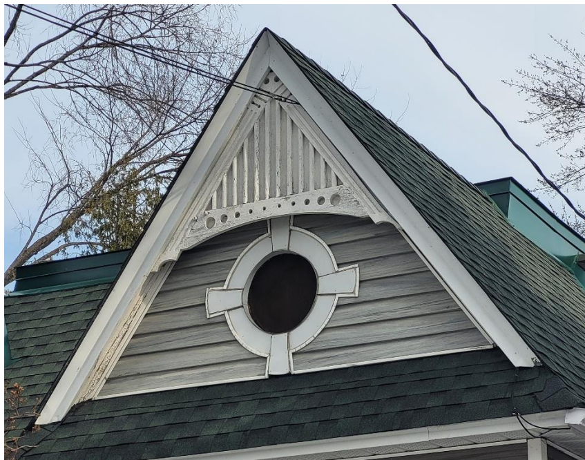
205 Bradford Street, southwest corner, front gable with millwork detailing and bull's eye window, Source: City of Ottawa, 2024
