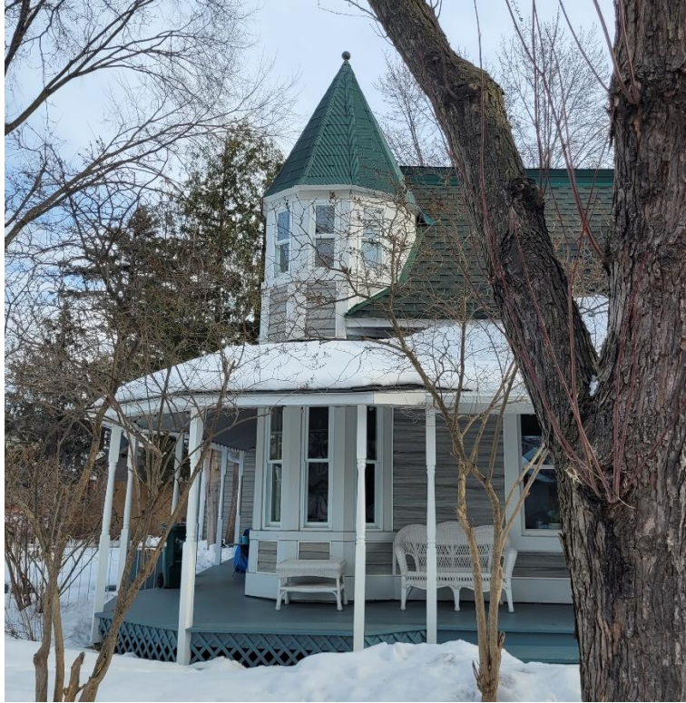
205 Bradford Street, northwest corner with turret, Source: City of Ottawa, 2024
