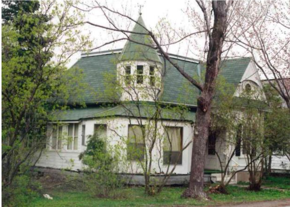
Northwest corner with turret and enclosed porch, 205 Bradford Street, Source: Horwitz and Tumak, Heritage Survey and Evaluation Form, 1996
