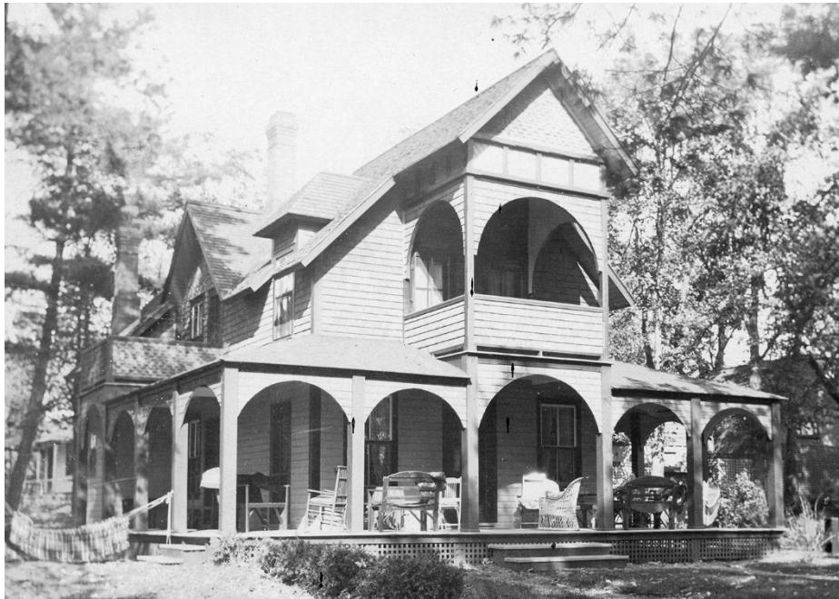
The Gables, dated 1905; 95 Kirby Road also built by Charles Robinson circa 1895, Source: City of Ottawa Archives, MG165-01-04, CA025471
