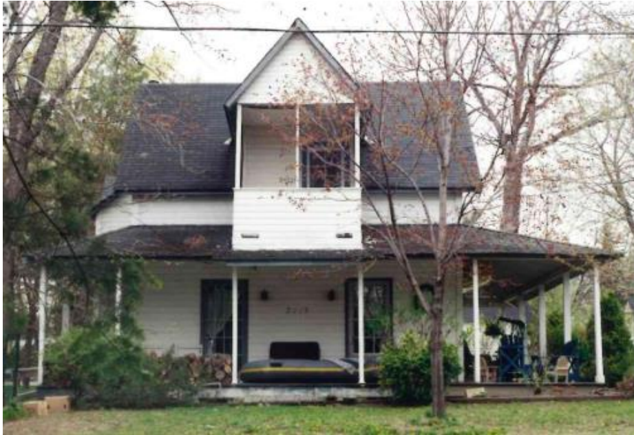
South façade, 2775 Rowatt Street, Source: City of Ottawa, L. Horwitz and E. Tumak, Heritage Survey and Evaluation Form, 1996
