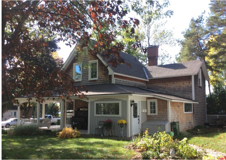
Northeast corner, 2775 Rowatt Street, Source: City of Ottawa, 2016
