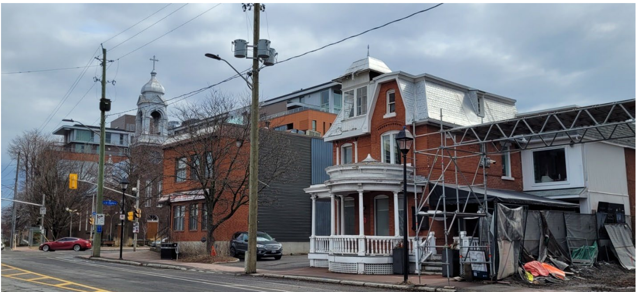
South side of Beechwood Avenue, looking east. St. Charles Church in background.
