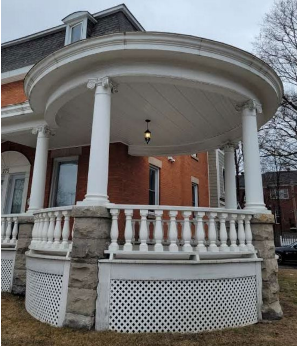
275 St. Laurent Boulevard, porch detail
