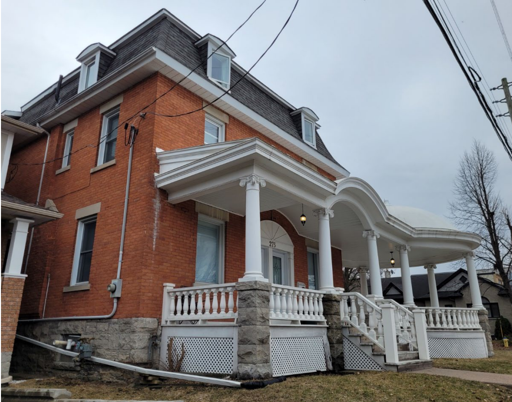
275 St. Laurent Boulevard, front façade (west)
