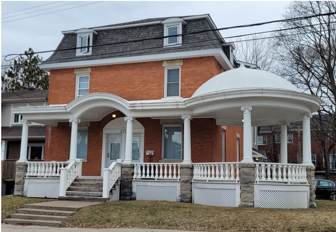
275 St. Laurent Boulevard, front façade (west)
