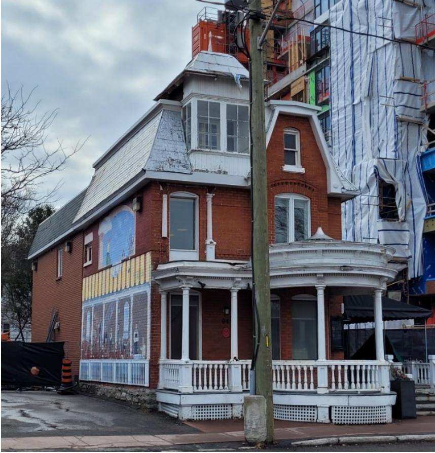
94 Beechwood Avenue, front façade (north)
