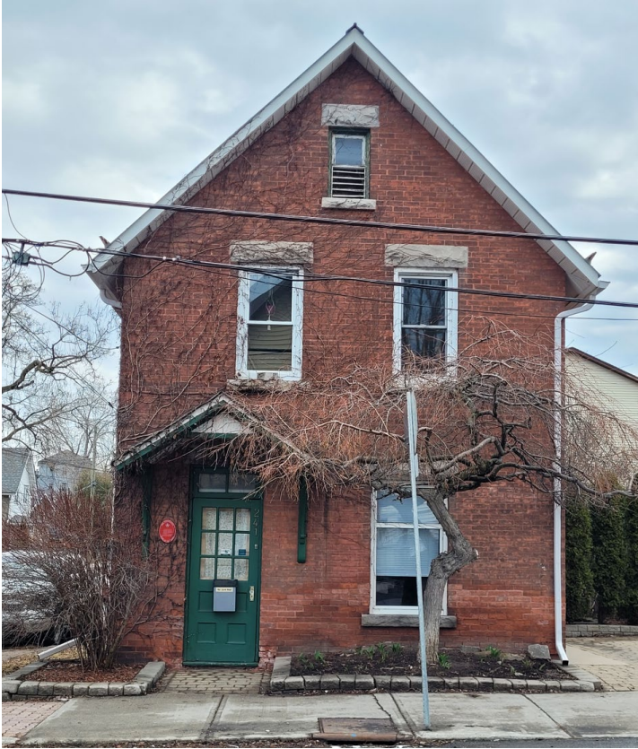
241 Marier Avenue, front façade (west)
