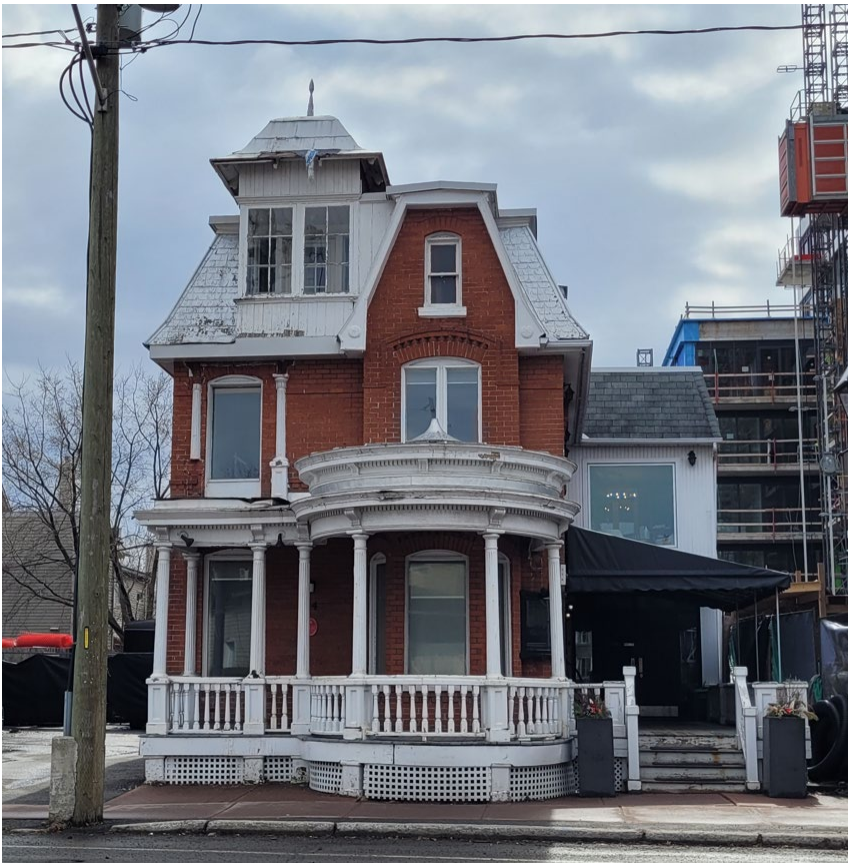
94 Beechwood Avenue, front façade (north)
