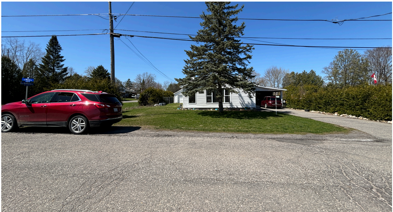
Figure 6: Across the street from the subject site on Mason Street
