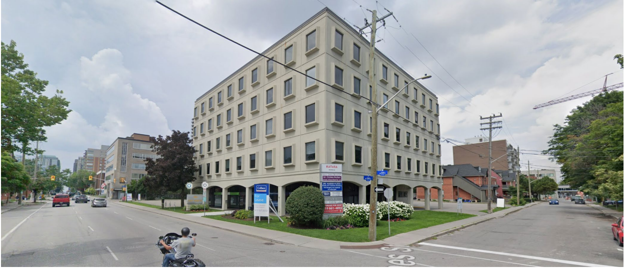
381 Kent Street, southwest corner. Google July 2023
