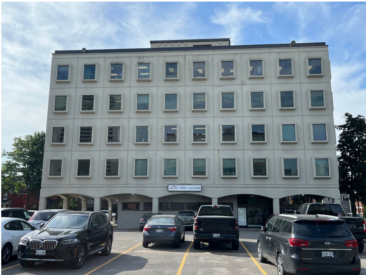
North façade of 381 Kent Street. June 2024
