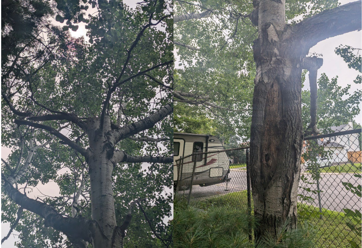
Above left: broken top and decay in Tree 1.
