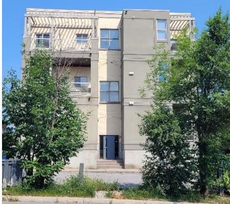
297 Dupuis Street, south façade, Source: City of Ottawa, 2024
