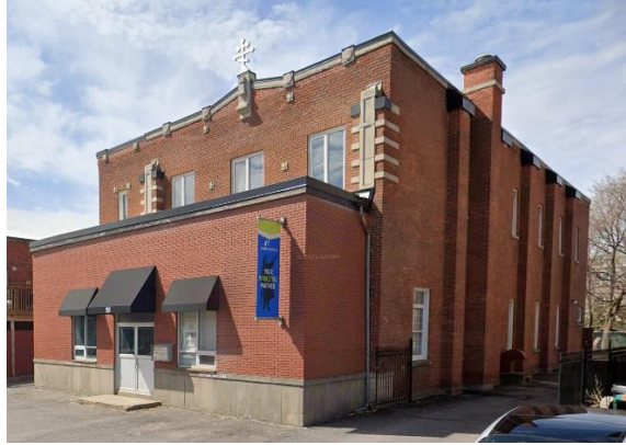
58 Arthur Street Street (1912), Source: Google Streetview, 2019
