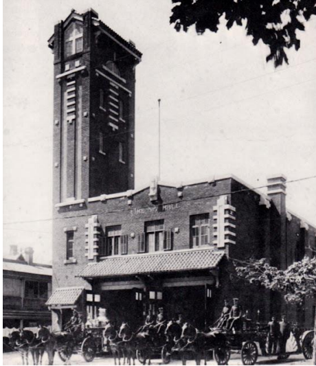
58 Arthur Street Street (1912), Source: Wilf Nelligan, https://urbsite.blogspot.com/2013/06/a-tale-of-two-francis-sullivan-buildings.html
