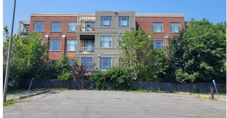
297 Dupuis Street, east façade, Source: City of Ottawa, 2024
