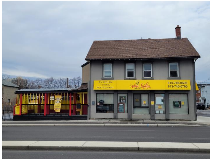
159 Montréal Road, south façade, Source: City of Ottawa, 2024
