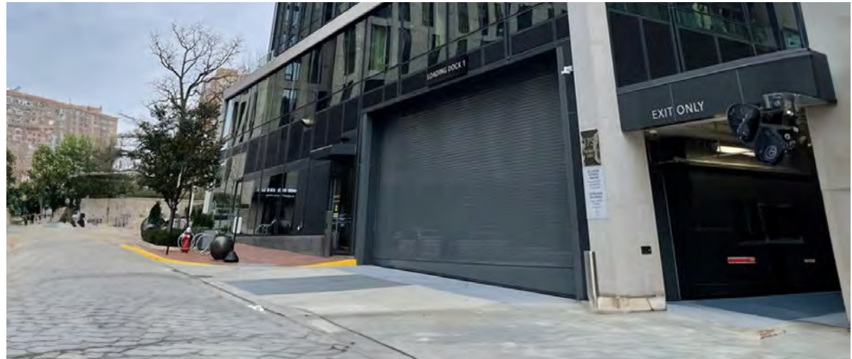
(Figure 4.5) This service entrance is off a private drive, integrates with the building style, and is adequately screened.
