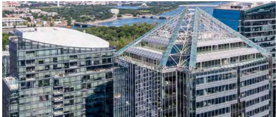
(Figure 3.9) The tops of buildings should make an overall contribution to the skyline of the KNED.
