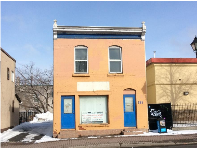
185 Montreal Street. Source: City of Ottawa.
