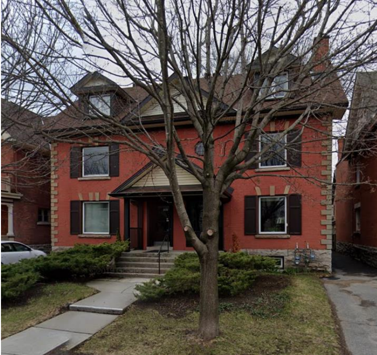
309 Stewart Avenue. Source: Google Street View, May 2019.
