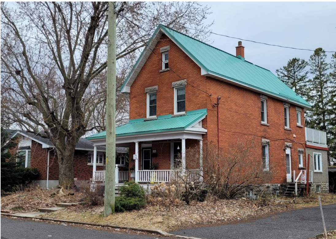
218 Cantin Street – Front façade (west)
