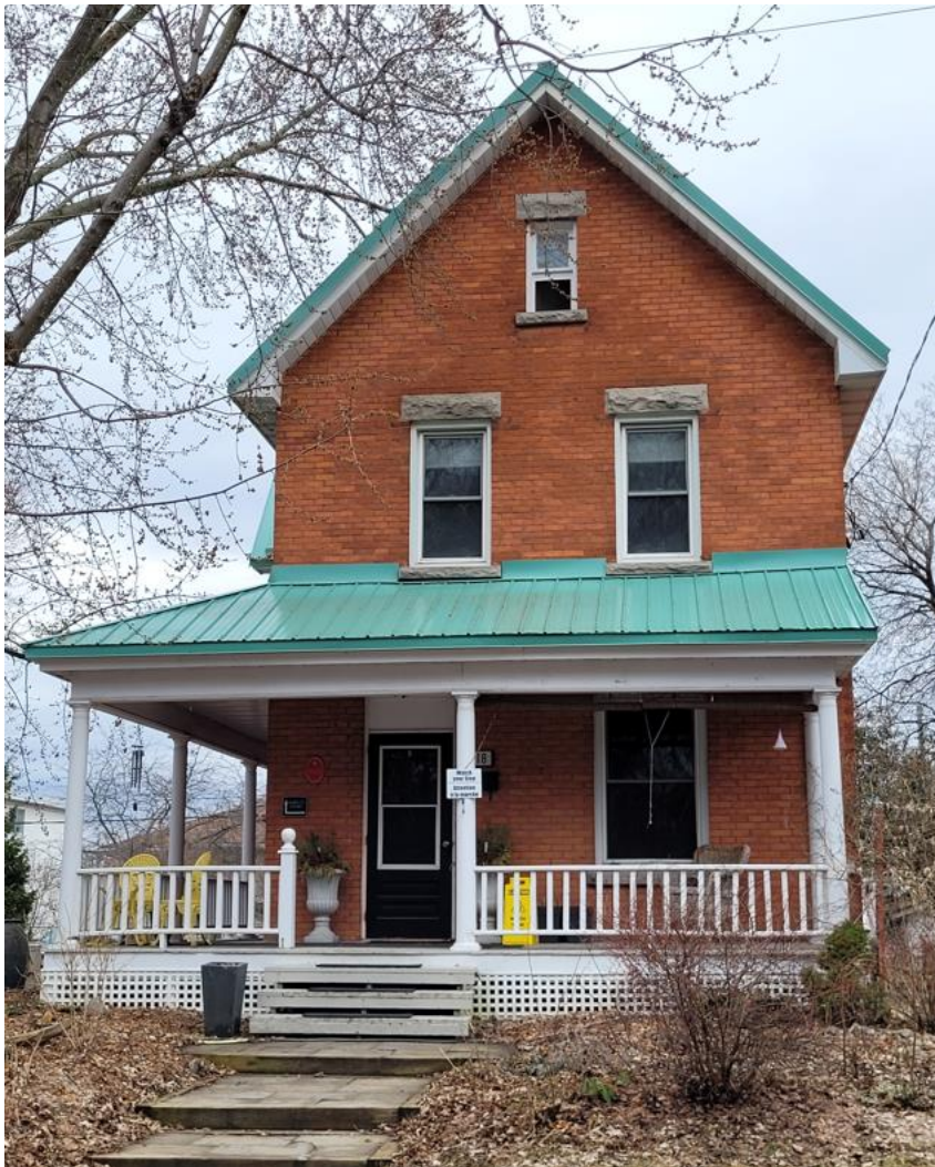
218 Cantin Street – Front façade (west)
