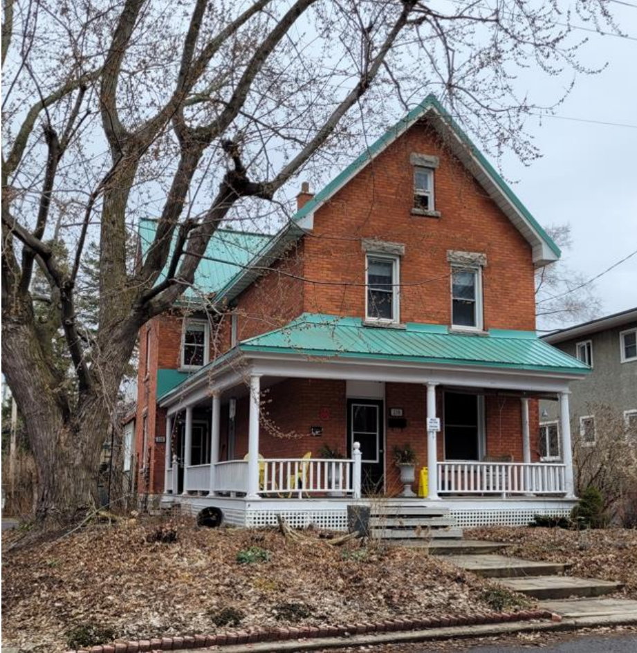
218 Cantin Street – Front façade (west)
