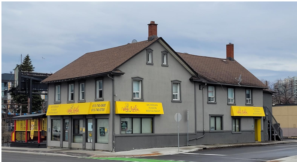
159 Montréal Road, southeast façade
