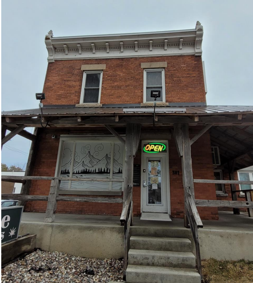
381 Montréal Road, front façade (south)
