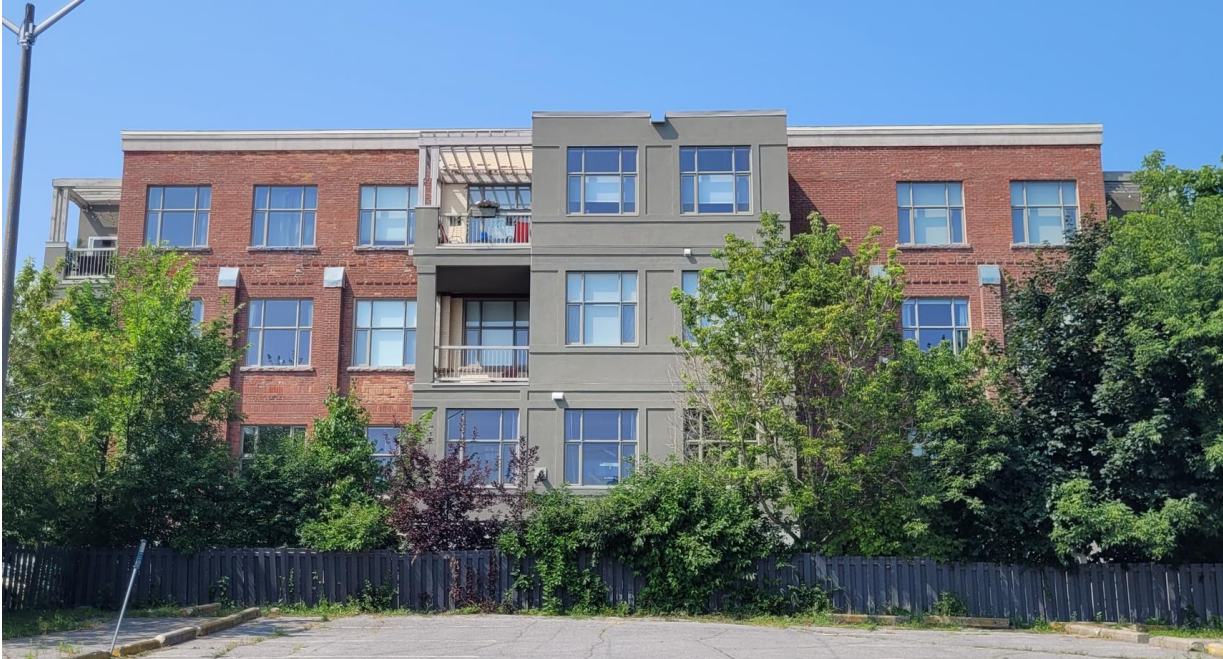
297 Dupuis Street, rear façade (east)
