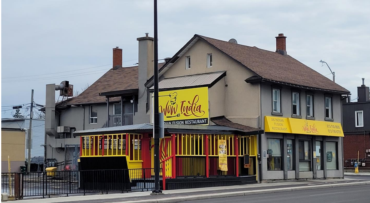
159 Montréal Road, southwest façade
