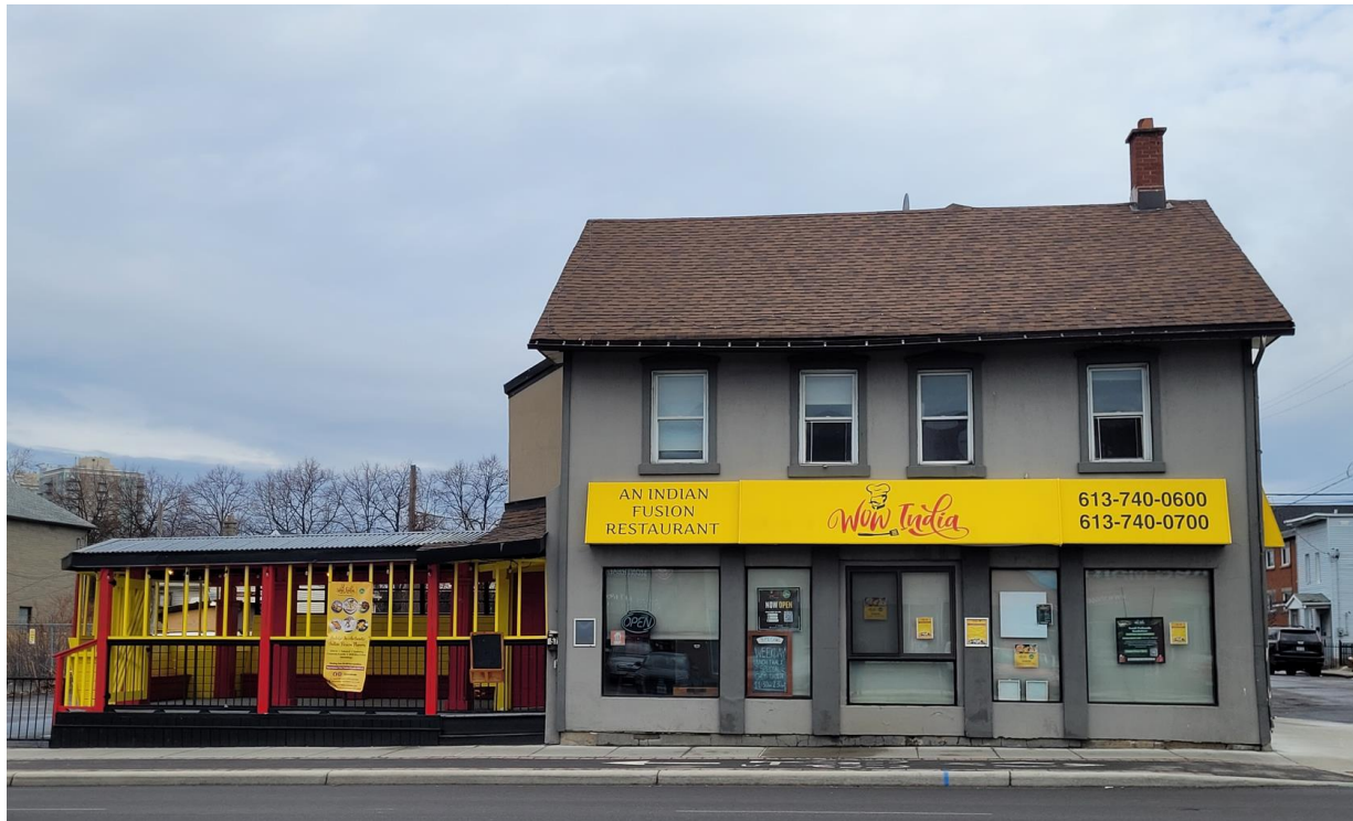
159 Montréal Road, front façade (south)
