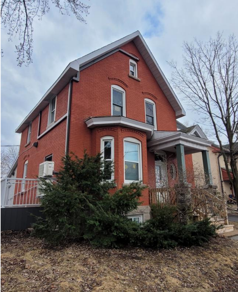
224 McArthur Avenue – Front façade (north)
