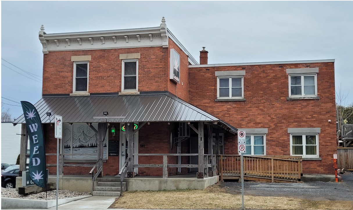
381 Montréal Road, front façade (south)
