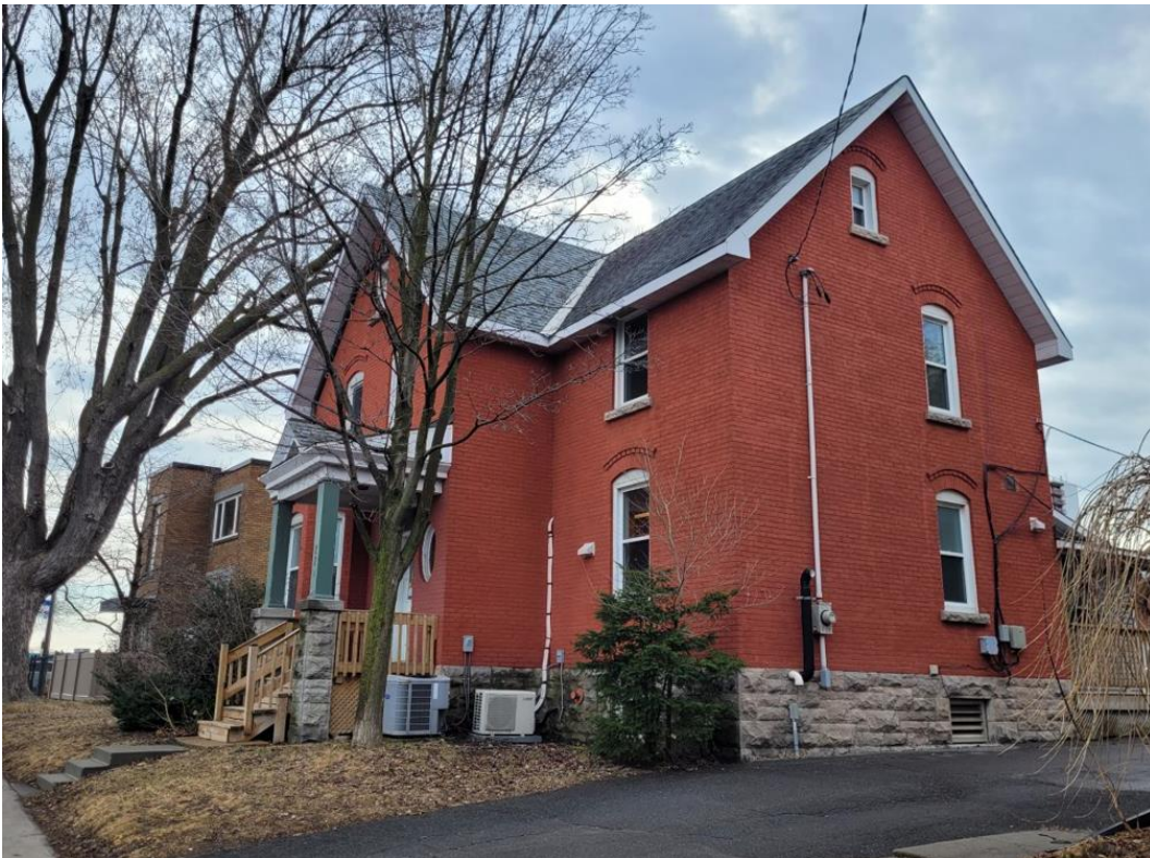
224 McArthur Avenue – Front façade (northwest)
