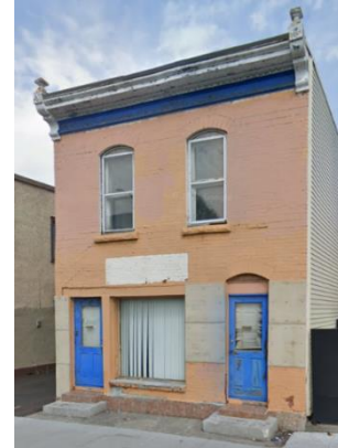
185 Montréal Road, Source: Google Street View, 2022
