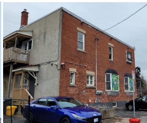
381 Montréal Road, west façade, Source: City of Ottawa, 2024
