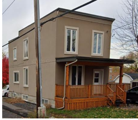
226 Alfred Street, Source: Google Street View, 2020
