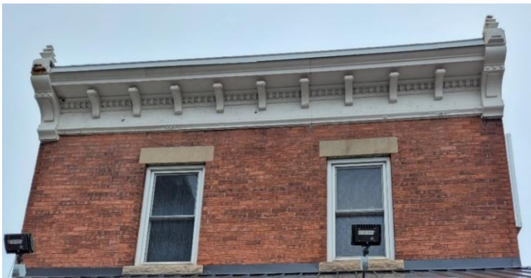
381 Montréal Road, cornice and stone lintels, Source: City of Ottawa, 2024
