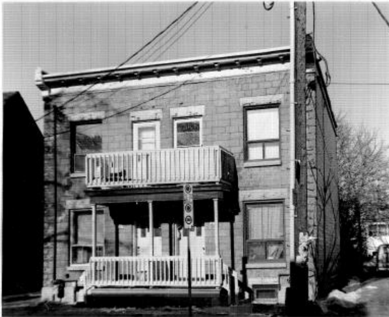
Attach building photos here: 1 - 6 x 6
