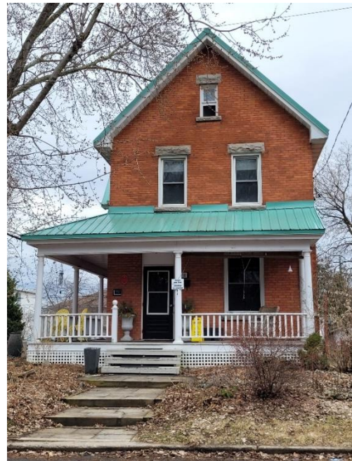
218 Cantin Street, front/east façade, Source: City of Ottawa, 2024
