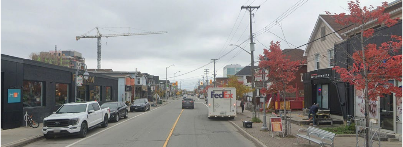
Figure 4: Street view looking north from the subject property on Preston Street.
