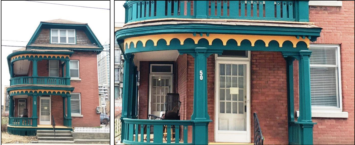
Cropped view of east façade (left) and detail of entry (right).
