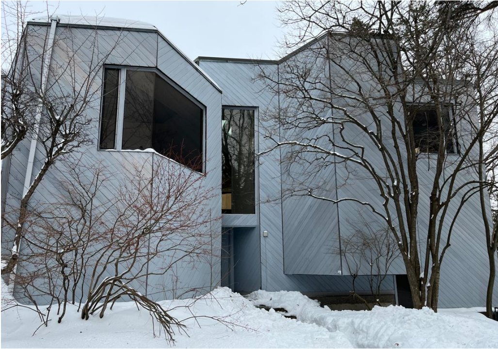
7 Crescent Road - Front façade, January 2023
