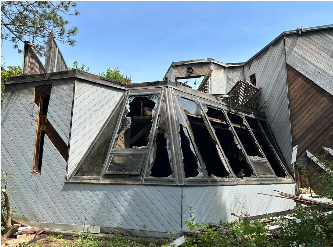
7 Crescent Road - Front façade, June 25, 2024
