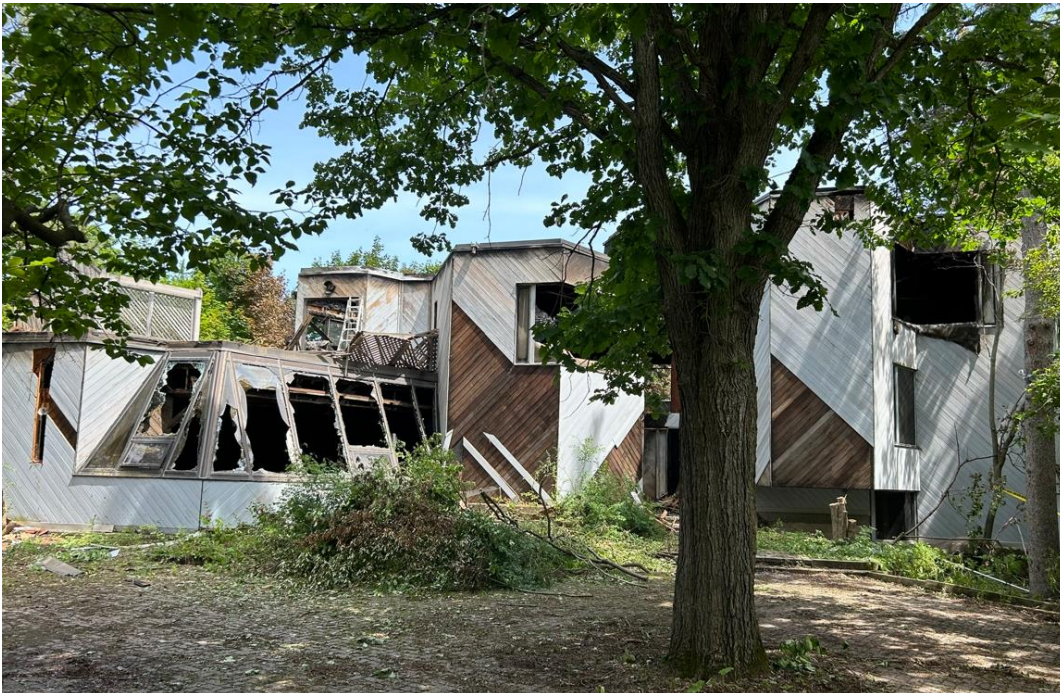
7 Crescent Road - Front façade, June 25, 2024
