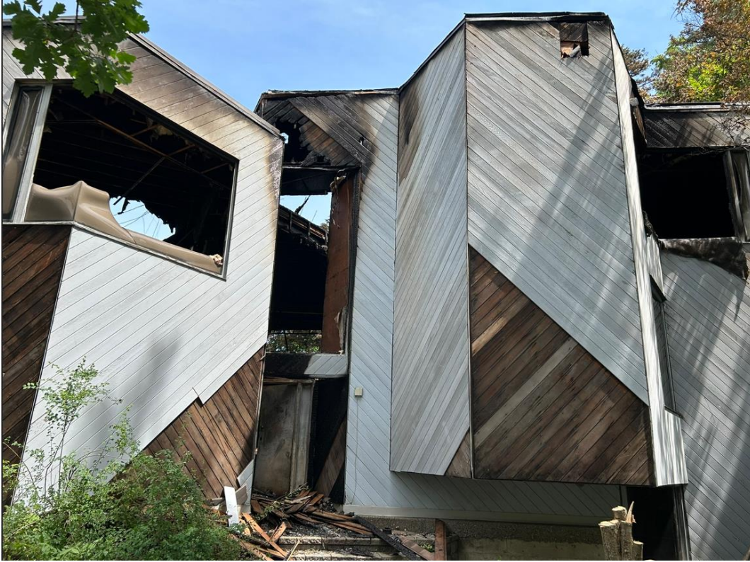
7 Crescent Road - Front façade, June 25, 2024
