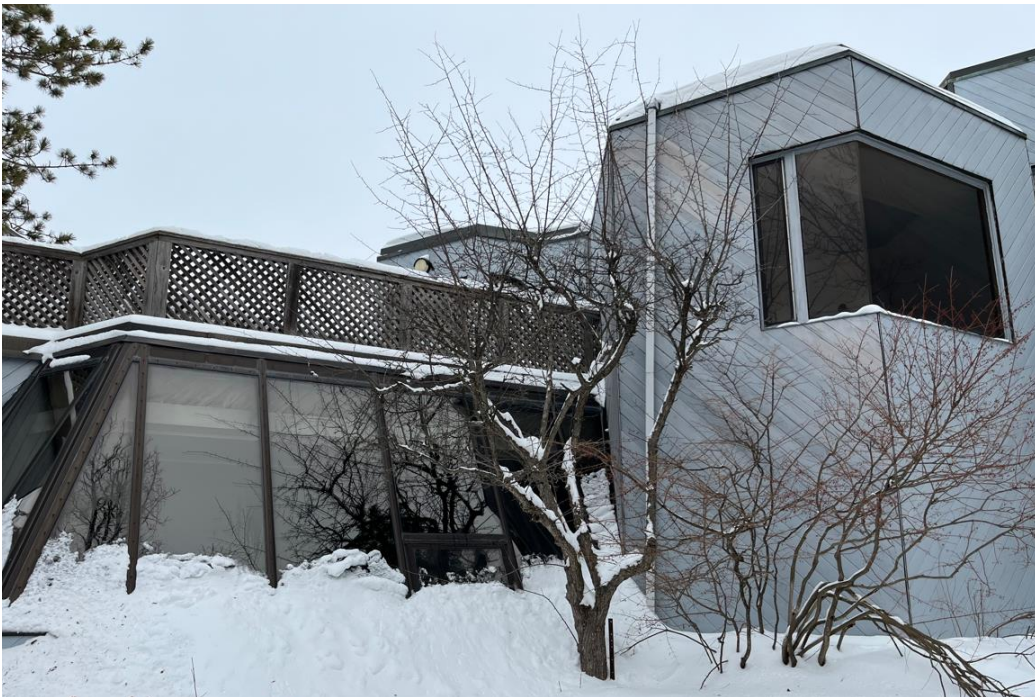
7 Crescent Road - Front façade, January 2023
