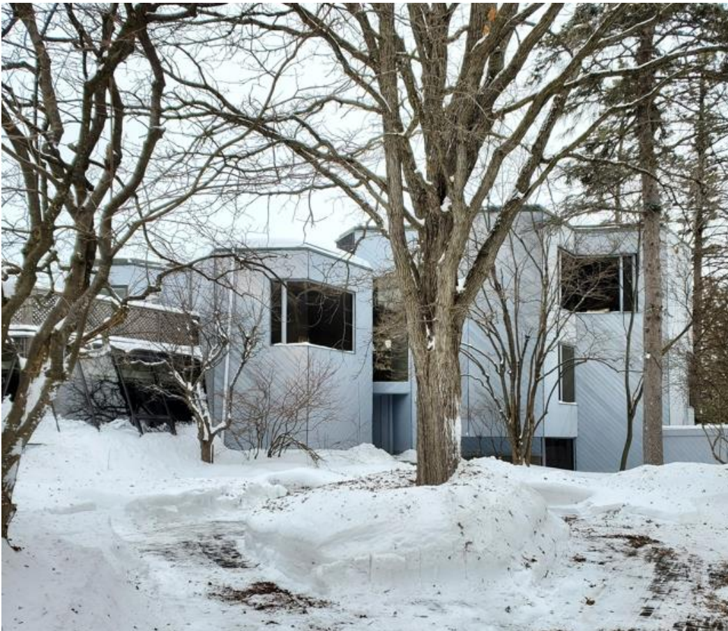
7 Crescent Road – Courtyard and front façade, January 2023
