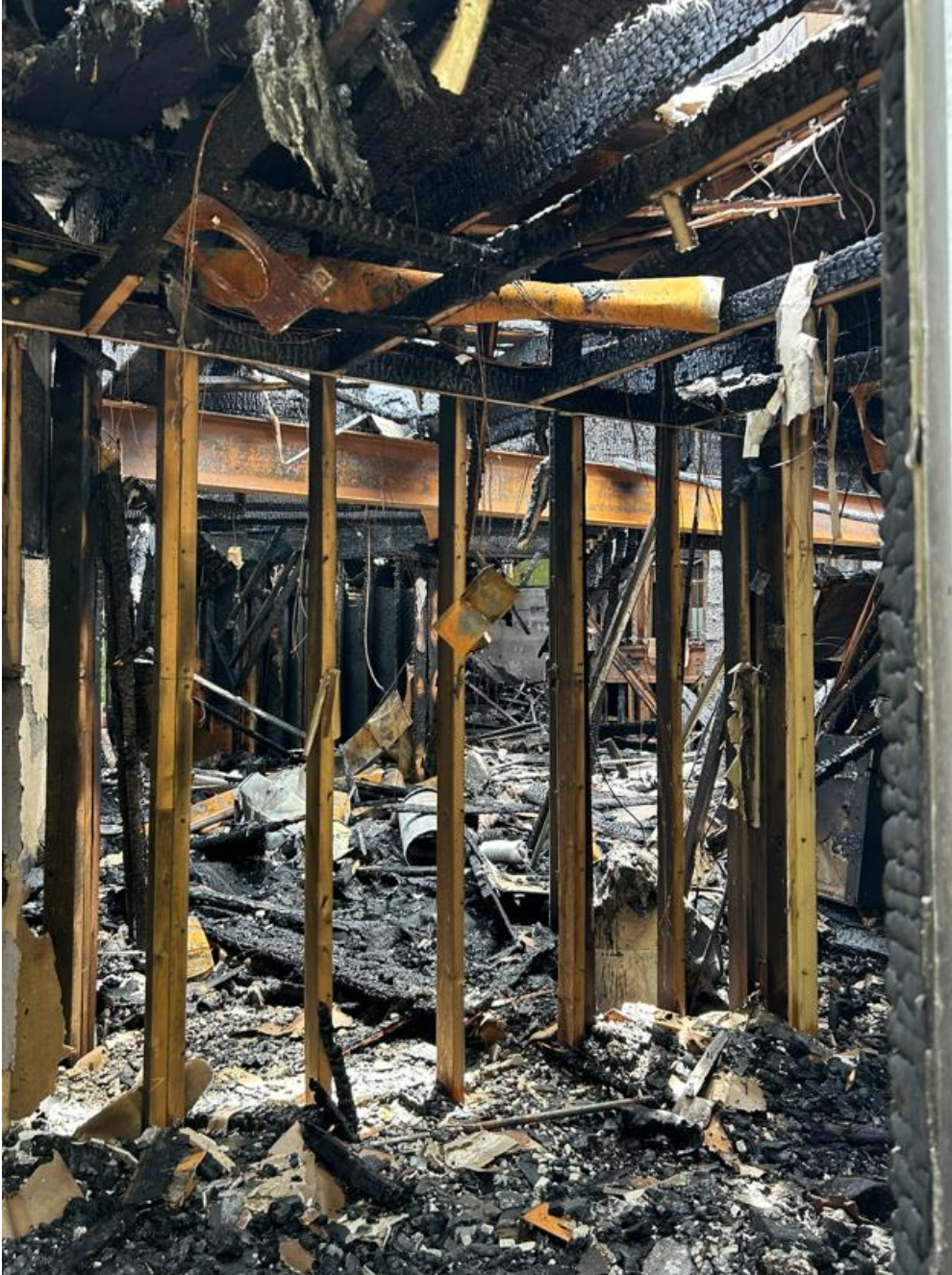
7 Crescent Road - Interior, June 25, 2024
