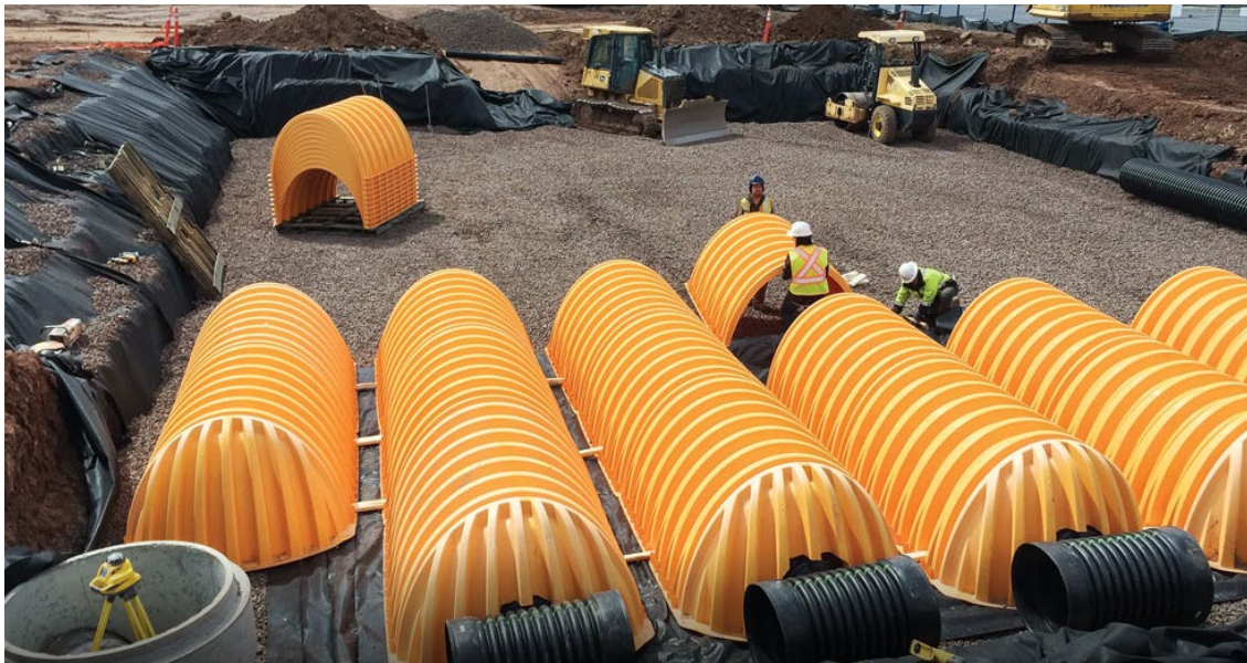
Figure 5.2. Underground Storage System, Courtesy Stormtech
