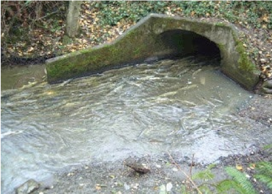
Figure 5.6. Creek Enclosure, Courtesy State of Washington
