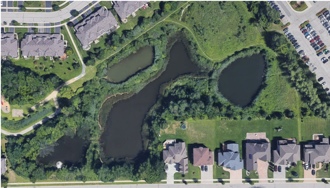
Figure 5.1. Krizsanderson Stormwater Management Facility, Kitchener, Designed by Wood
