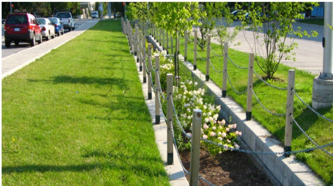
Figure 5.3. Bioretention System, Courtesy Sustainable Technologies
