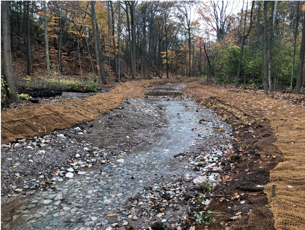
Figure 5.4. Creek Realignment, Post Construction, West Morrison Creek
