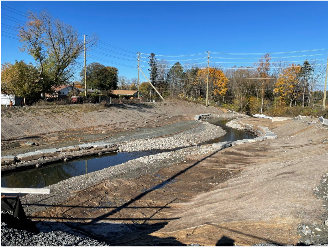
Figure 5.8. Channel Hardening using Armour Stone and Riprap
