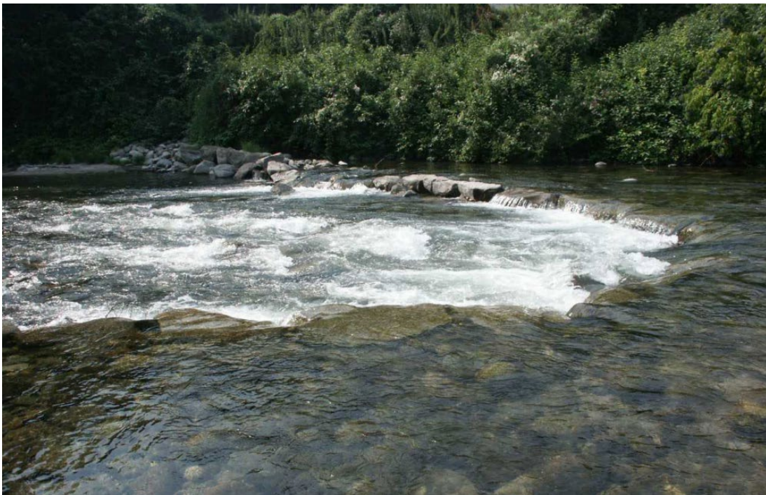
Figure 5.18. Cross Vane, Courtesy Coldwater Consulting
