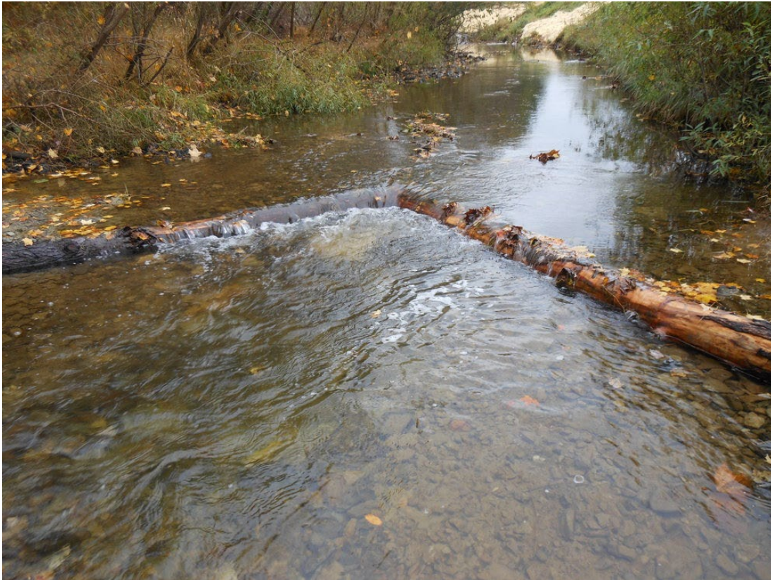
Figure 5.17. Log Weir, Courtesy Cambria County Conservation
