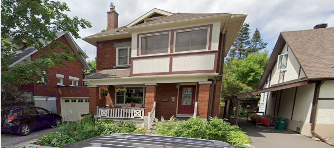
Image 1. View of existing Front elevation along Bower St
