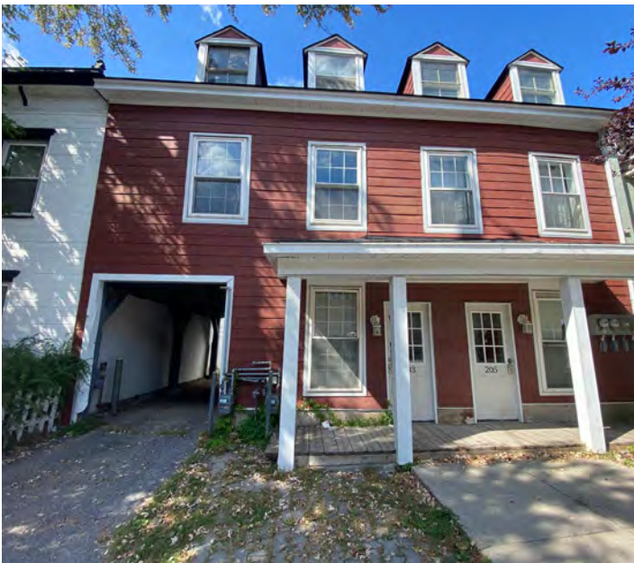
Figure 42: Carriageway on Bruyère Street.
