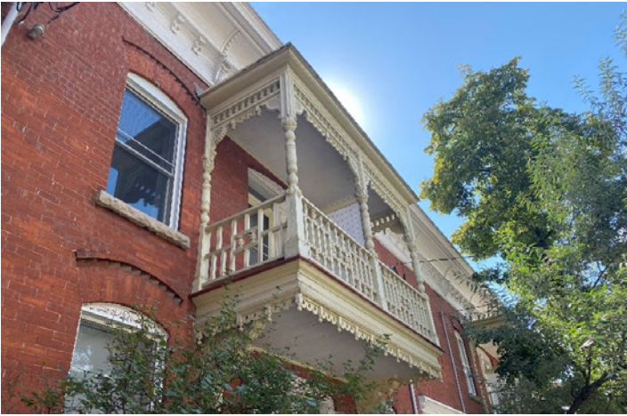
Figure 41: Cantilevered balcony at 208 St. Patrick Street.
