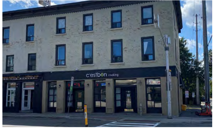
Figure 36: Storefronts on Dalhousie.
