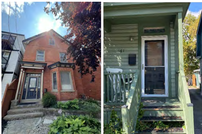
Figure 39: Examples of doors in the HCD.
