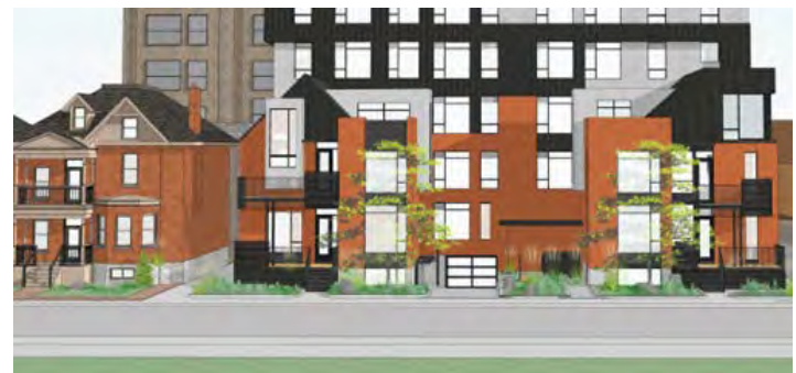
Figure 26: Example of an infill project to construct a mid-rise building and two contemporary houses at the street, incorporating the mass, forms, height and details from other buildings in the streetscape (porches, roof styles, setbacks etc.) Credit: Colizza Bruni Architecture.
