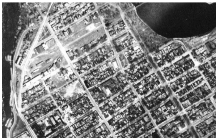
Figure 6: Aerial image of Lowertown, 1928. Retrieved from GeoOttawa.ca.
