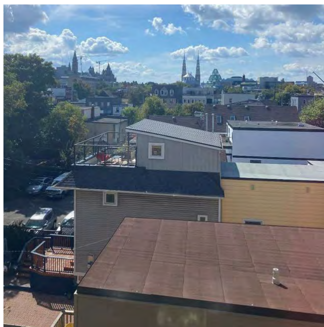
Figure 45: Example of roof top addition at the rear of a property.
