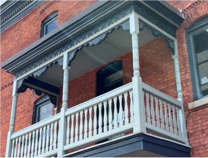
Figure 35: Balcony with decorative trim.
