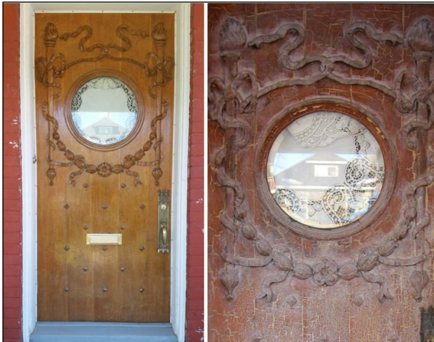
Carvings on the oak front door with circular window insert. Source: Current property owner.
