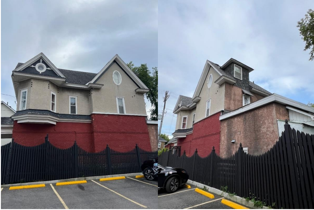
North façade, with one-storey timber section clad in stucco attached at the rear northwest corner. Source: City of Ottawa, August 2024.
