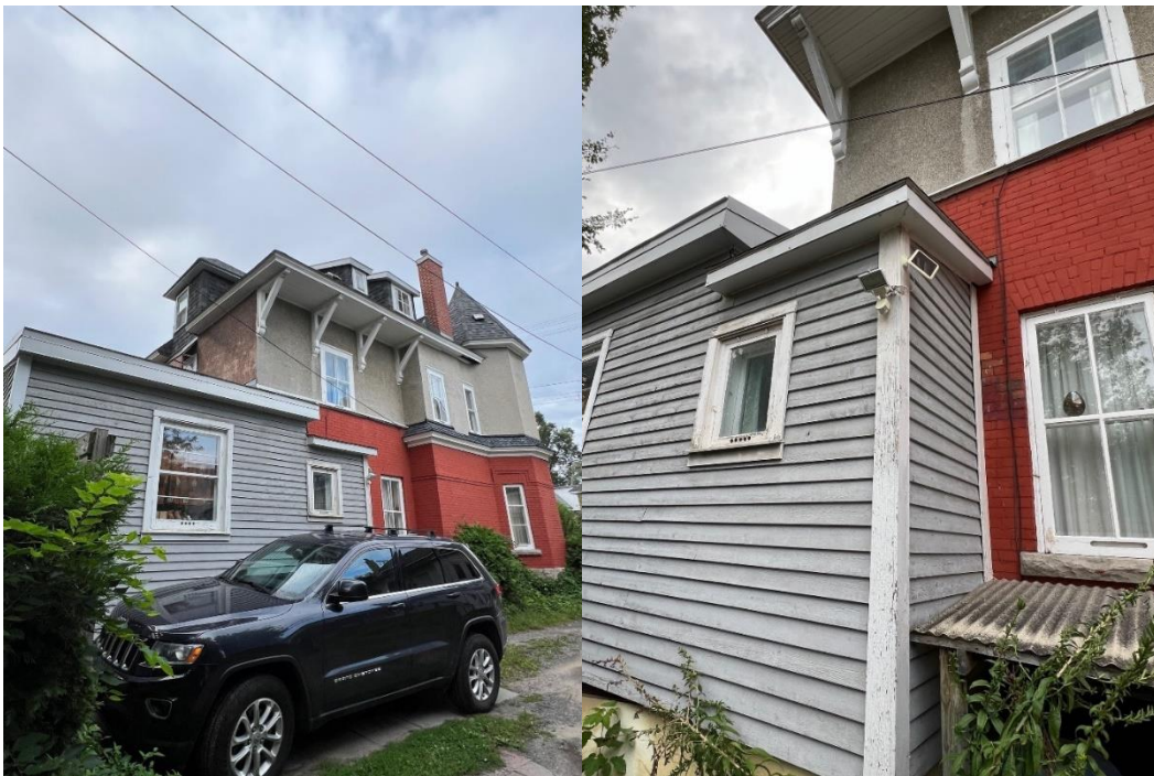
South elevation with addition from the 1950s, clad in grey cedar siding, attached at the rear southwest corner. Source: City of Ottawa, August 2024.
