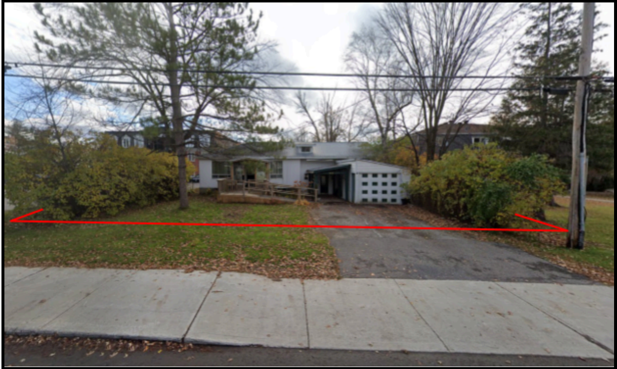
2458 Cleroux from Cleroux Cres showing the approximate location of the lot lines.
