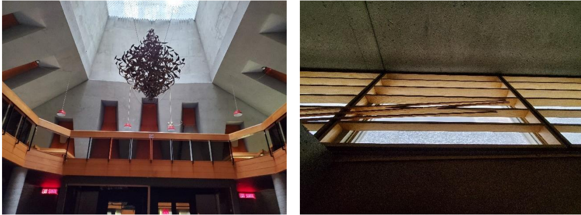
(L-R) Figure 5A: Pavilion A interior showing the lightwell at the top of the pyramidal roof, reflecting light onto sculpture; Figure 5B: Pavilion A interior showing glass soffits (City of Ottawa, 2021).
