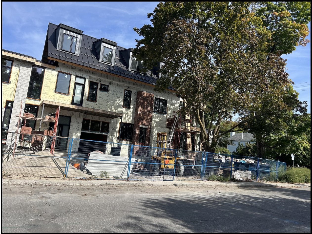
Subject property Dovercourt frontage. September 2023 photo. Construction nearing completion
