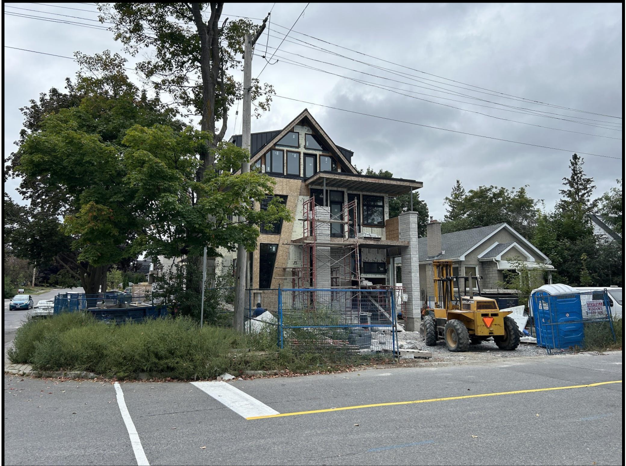
Subject property Tweedsmuir frontage. September 2023 photo. Construction nearing completion
