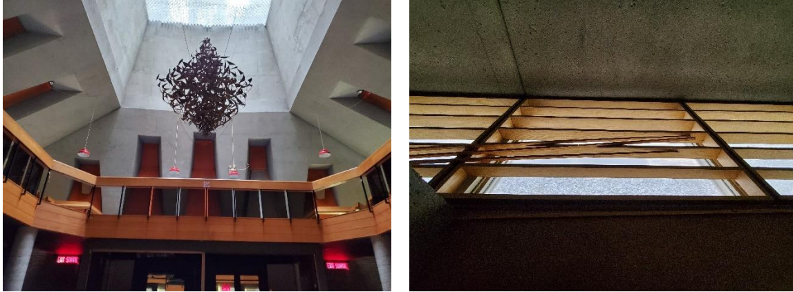
(L-R) Figure 5A: Pavilion A interior showing the lightwell at the top of the pyramidal roof, reflecting light onto sculpture; Figure 5B: Pavilion A interior showing glass soffits (City of Ottawa, 2021).
