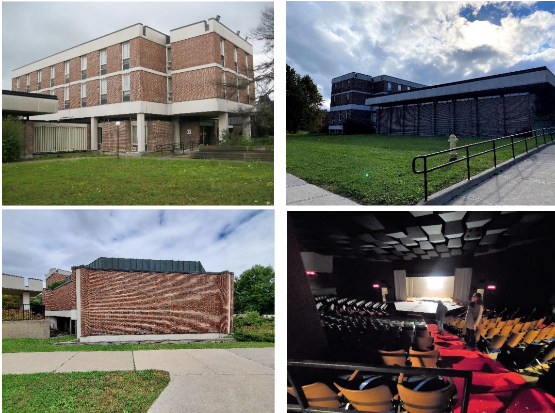
(L-R) Figure 8A: Pavilion E from the central quadrangle (City of Ottawa, 2013); Figure 8B: Pavilion E from the central quadrangle; Figure 8C: Pavilion F front exterior elevation; Figure 8D: Pavilion F interior (City of Ottawa, 2021).
