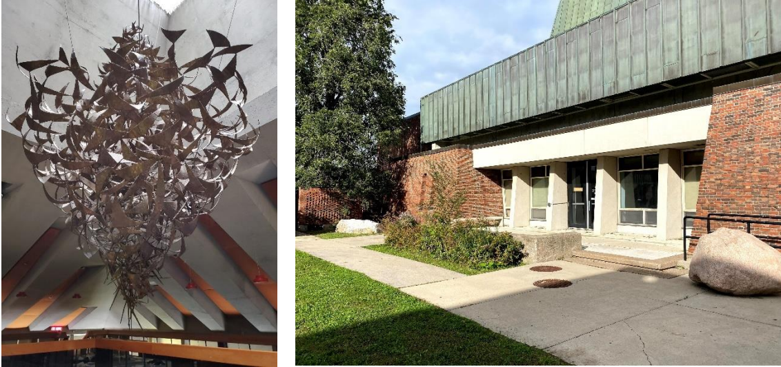
(L-R) Figure 11A: “Christ With Manna From Heaven” light sculpture; Figure 11B: Pavilion A west elevation demonstrating concrete banding and copper roof (City of Ottawa, 2021).
