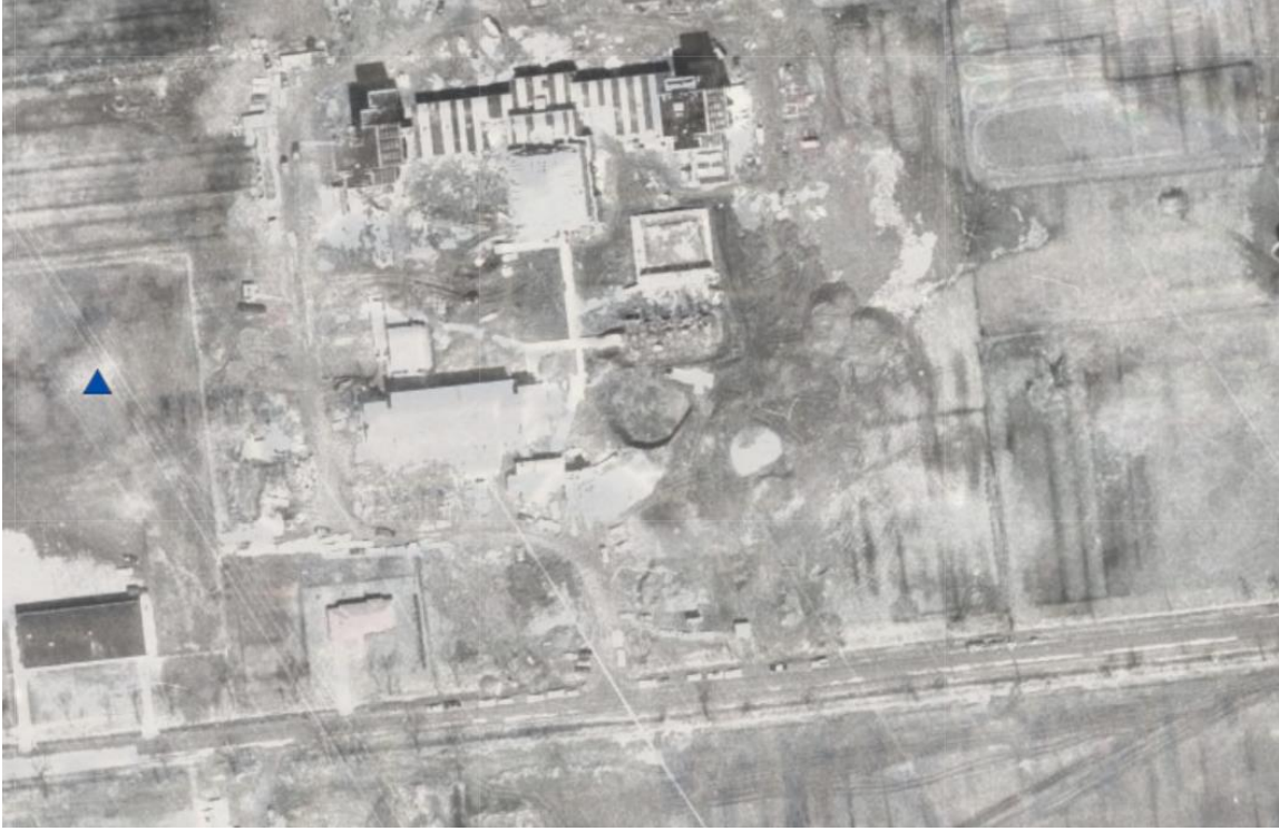
Figure 14: Aerial view of Campanile in 1963, during construction (City of Ottawa, 2022).
