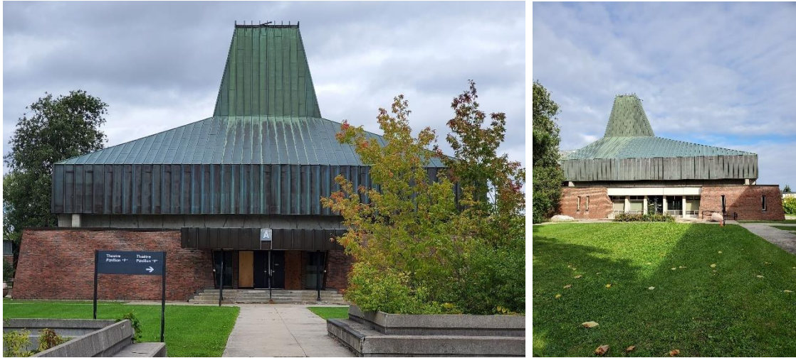
(L-R) Figure 4A: Front elevation of Pavilion A; Figure 4B: Side (west) elevation of Pavilion A (City of Ottawa, 2021)
