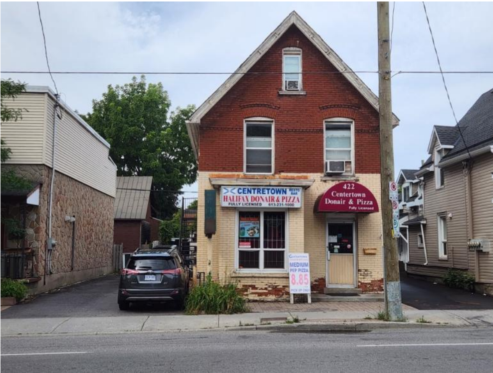
422 BRONSON AVE. – EAST FACING STREETSCAPE
