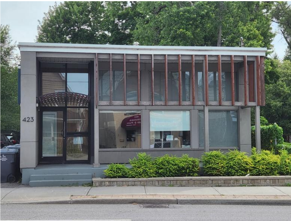
423 BRONSON AVE. – WEST FACING STREETScape
