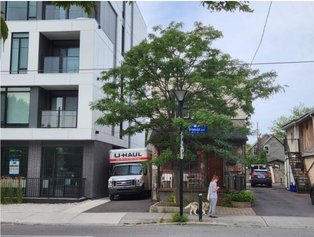
444 BRONSON AVE. – EAST FACING STREETScape
