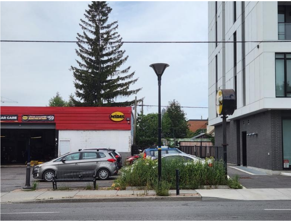
448-450 BRONSON AVE. – EAST FACING STREETScape
