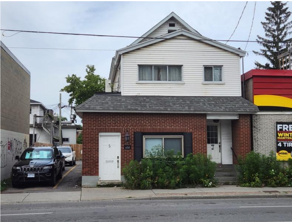
456 BRONSON AVE. – EAST FACING STREETScape
