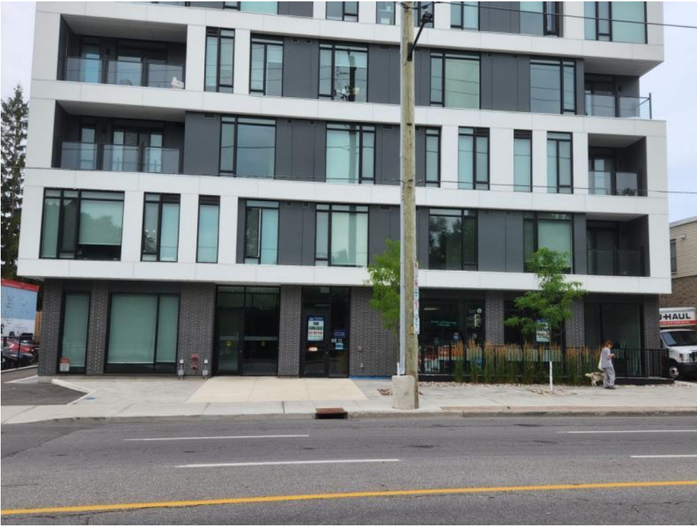
444 BRONSON AVE. – EAST FACING STREETScape
