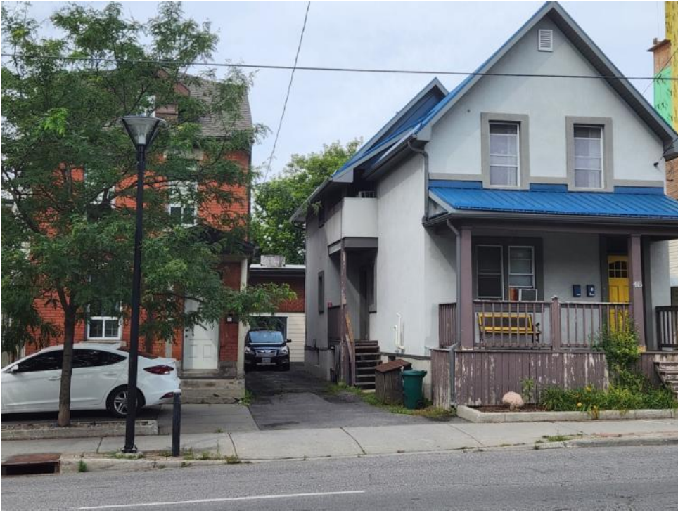
418 BRONSON AVE. – EAST FACING STREETScape
