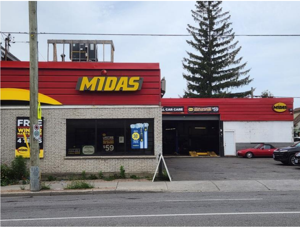
448-450 BRONSON AVE. – EAST FACING STREETScape
