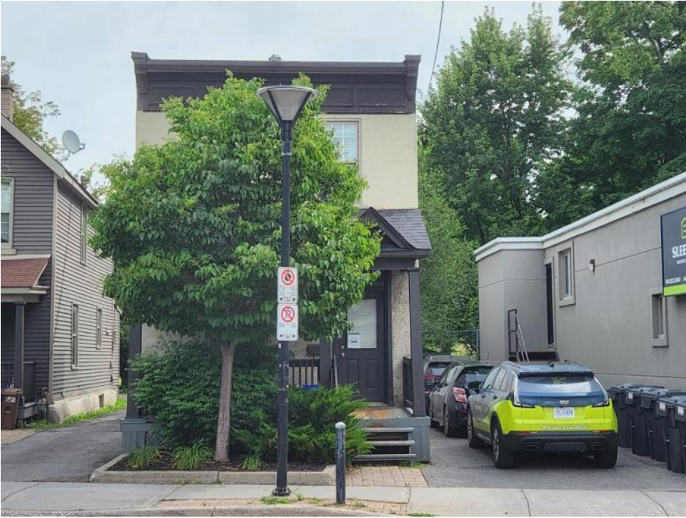
421 BRONSON AVE. – WEST FACING STREETScape
