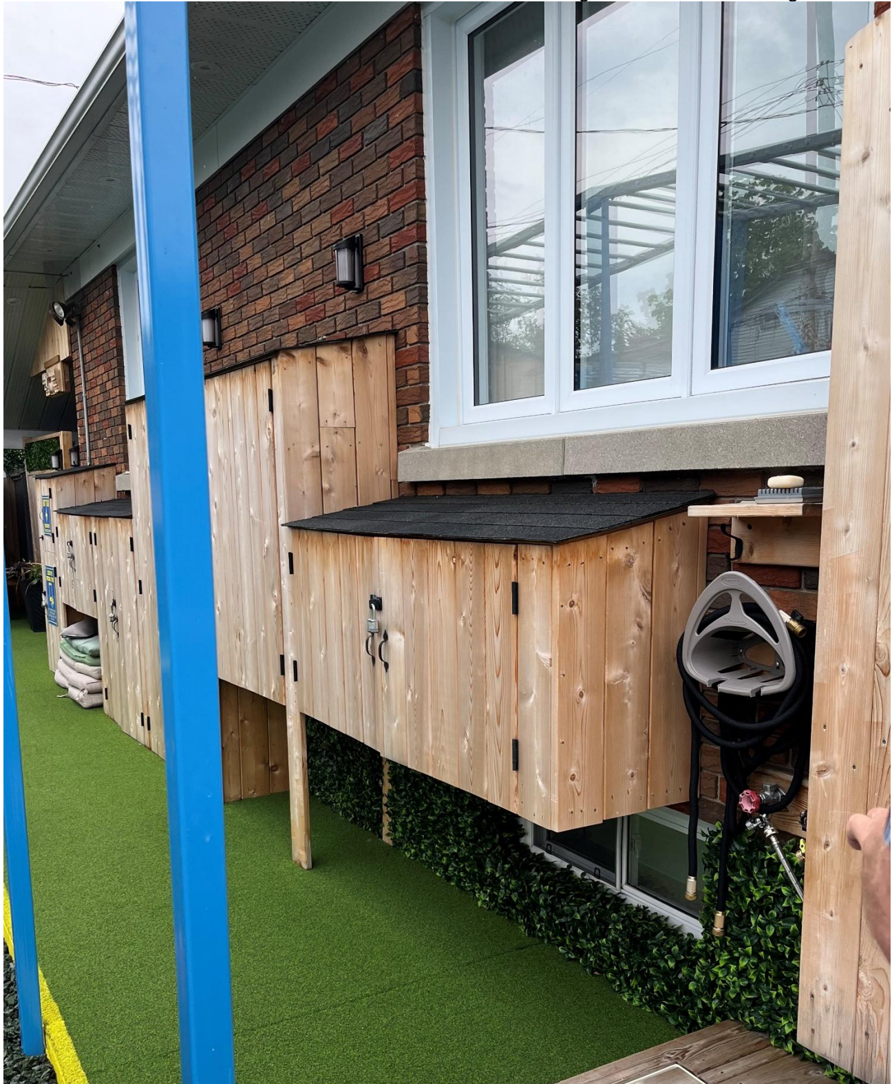
Figure 15: Wooden Storage Lockers.
