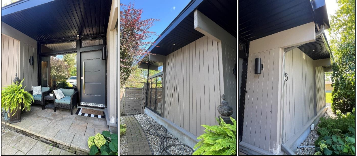
Photos 7-9: Front (north) façade.
