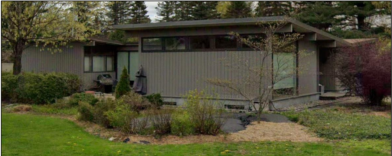
East elevation at 8 Robert Kemp Street in 2019. Source: Google Street View, May 2019.
