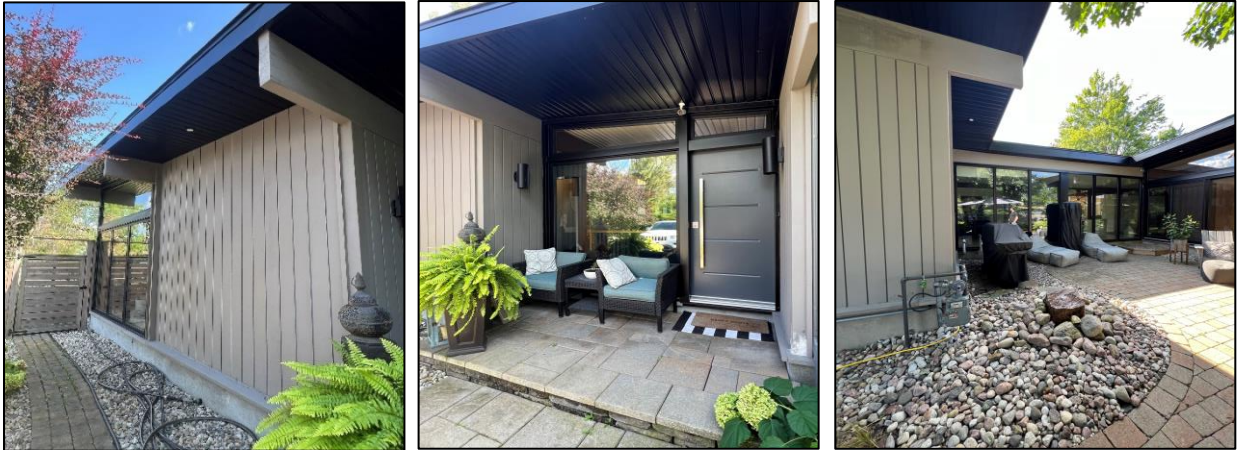
Vertical wood siding, exposed wood beams, recessed entrance, large windows, and clerestory windows at 8 Robert Kemp Street. Source: City of Ottawa, 2024.
