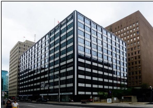
The Fuller office building by Balharrie, Helmer & Morin, 1961-62. Source: Rick MacEwan, 2014.
