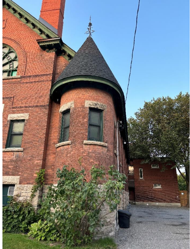
The church's turret on the west façade. City of Ottawa, 2024.
