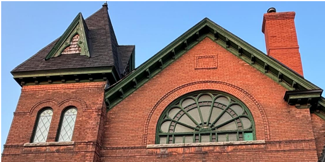
The church's front façade featuring a decorative brick stringcourses and bandings, a half-round rose window with wooden tracery and coloured glass, date stone, and decorative wooden soffits. City of Ottawa, 2024.
