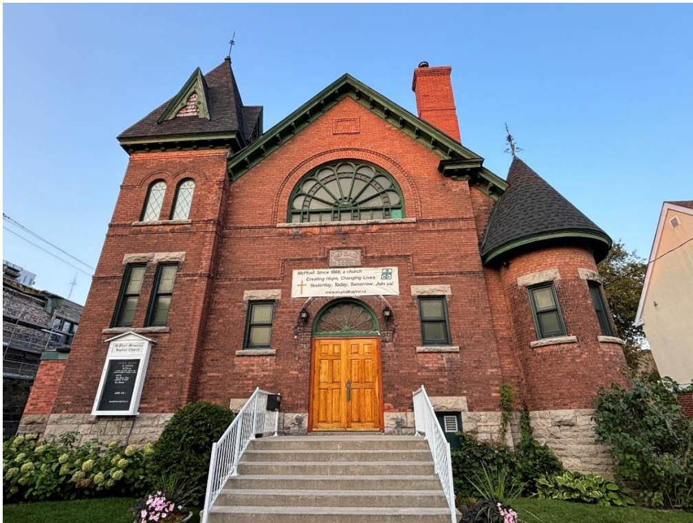
The McPhail Memorial Baptist Church's front façade on Bronson Street. City of Ottawa , 2024.
