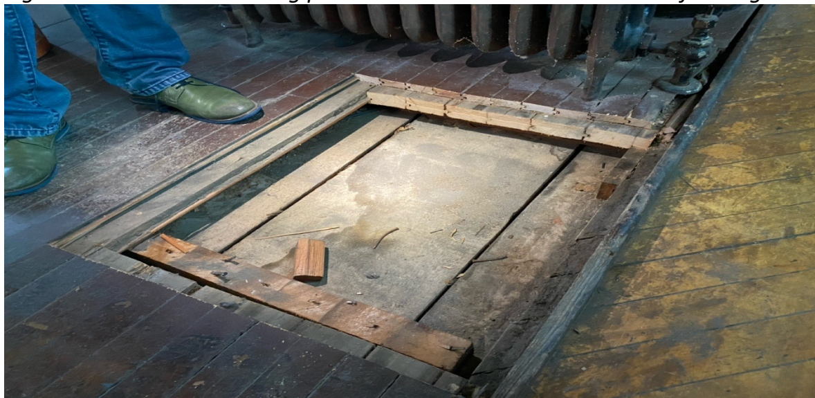
Figure 10). Exploratory opening showing construction detail of raised hardwood flooring.
