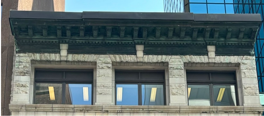
Fifth storey and roofline featuring copper architrave, frieze, and cornice. City of Ottawa, 2024.
