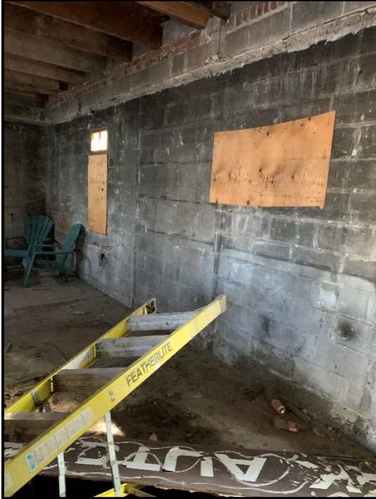
Exposed Masonry Wall Administration Area
