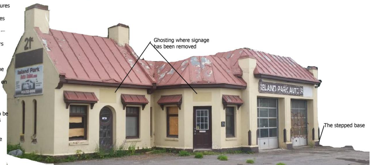
Figure 4: Annotated view of the Service Station highlighting the identified attributes. Source: Commonwealth
