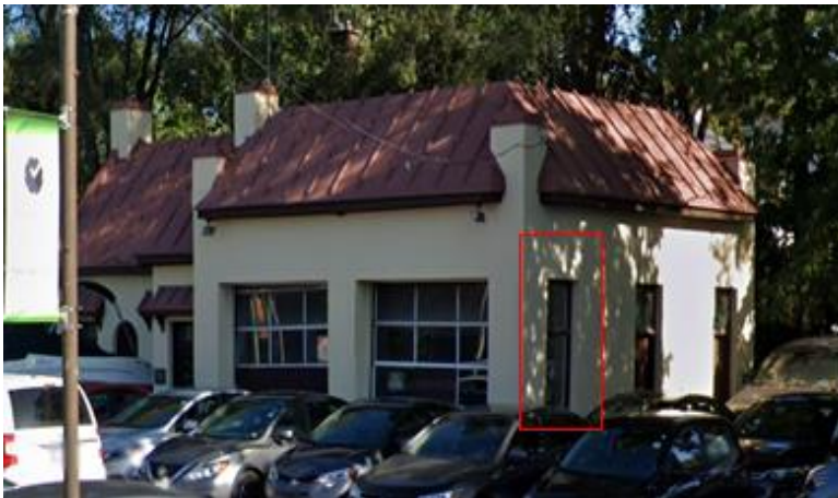
Figure13: This view highlights in red the first of the three windows along the west side of the Service Station. The proposed midrise building has been set back and allows one of the side windows to be interpreted from the exterior and the others will be incorporated into the lobby entrance. Source: City of Ottawa.
