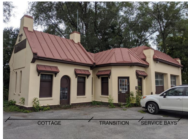
Figure 1: View of the Service Station with the 3 sections cottage, transition, and service bays.
