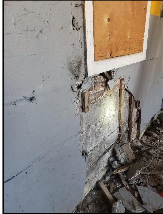
Masonry Wall Behind Plaster Lath - Service Bay
