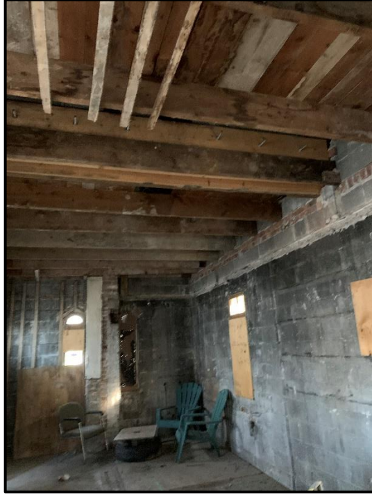
Roof framing administration area
