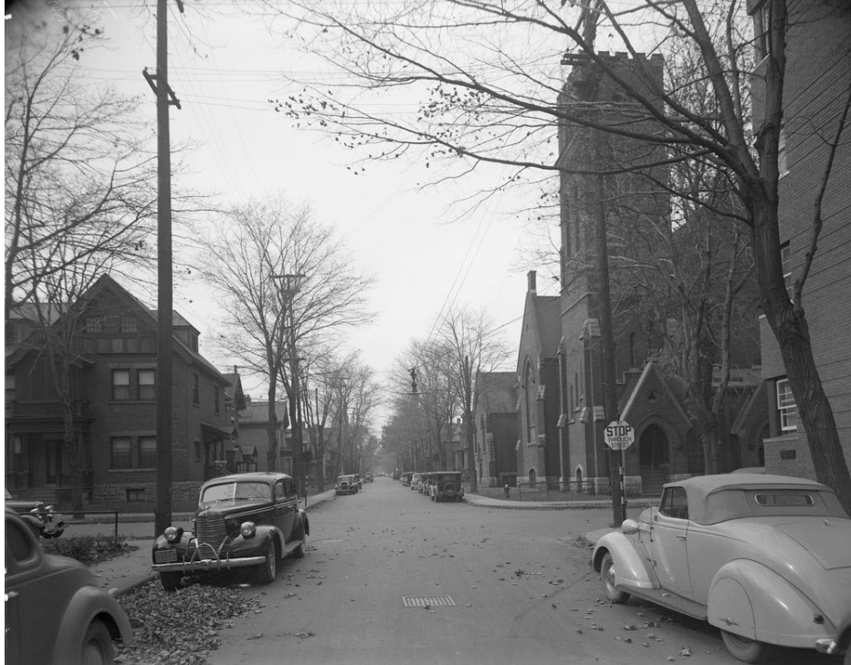
Metcalfe and Gloucester Street, n.d. Canada Department of Public Works 1979-140 NPC, RV1 038 4170144, Library and Archives Canada .
