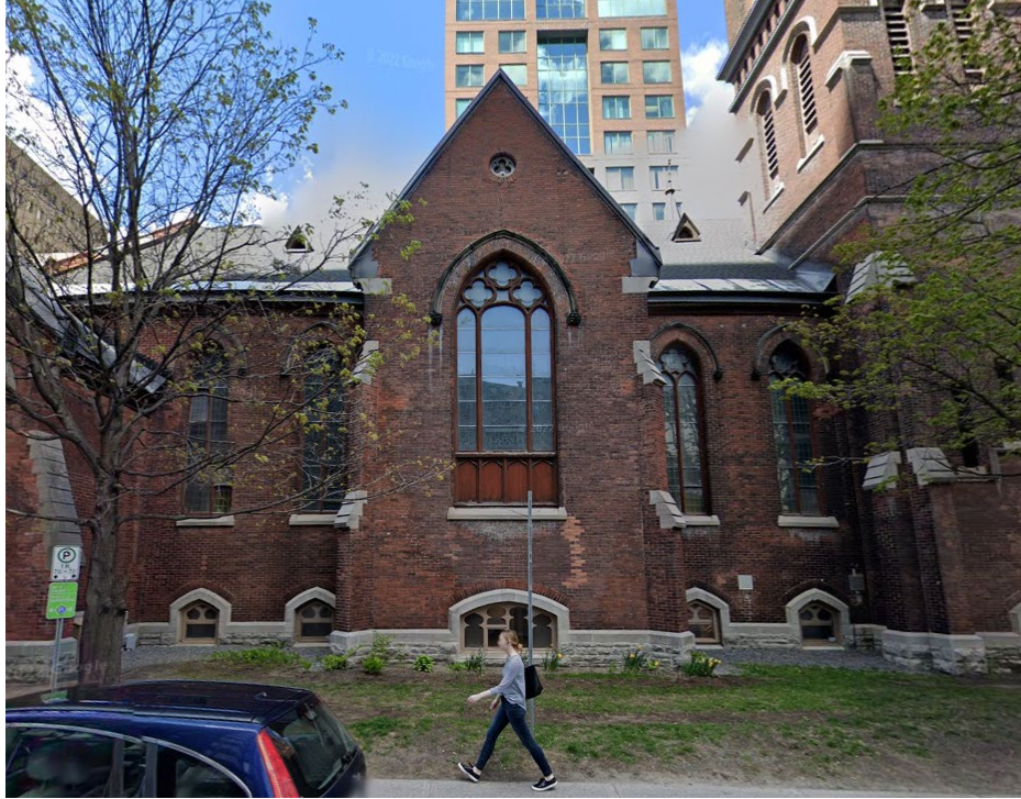
Gloucester Street façade, Google Maps , 2021.
