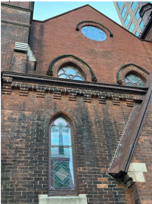
Metcalf Street façade showing decorative brickwork, coloured, and stained-glass windows.
