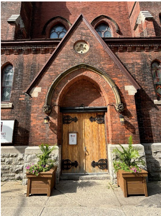
Main entrance on Metcalfe Street showing carved stone trefoil, hood moldings and label stops. City of Ottawa, 2024.
