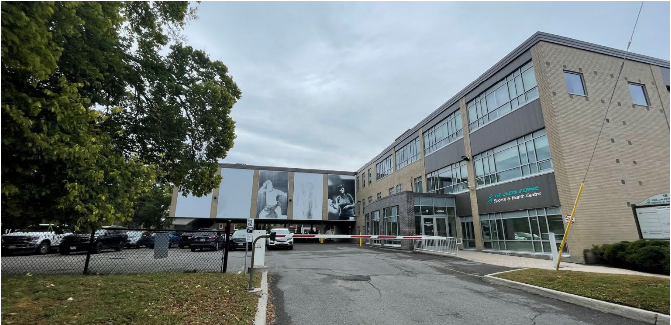
Figure 6. View of the existing building and site access from Louisa Street
