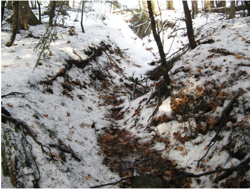
Photo 26 – Location of emergency spillway looking north towards top of valley slope from north of the South Tributary (December 16, 2021)
