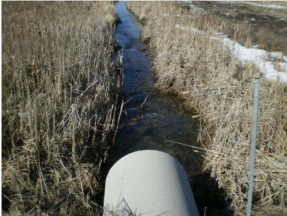
Photo 1 - South tributary looking west from culvert under Cox Country Road (March 17 th , 2020)
