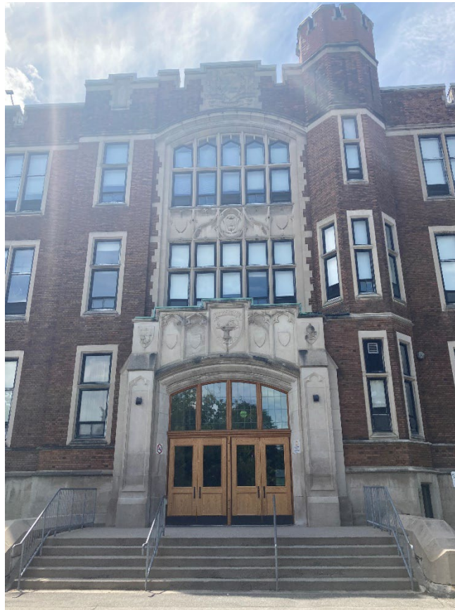
Glebe Collegiate Institute, front entrance facing Percy Street (City of Ottawa, 2022)
