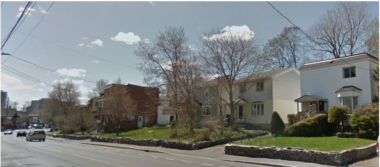
View looking west on Beechwood showing the subject properties (Google Streetview, 2016)
