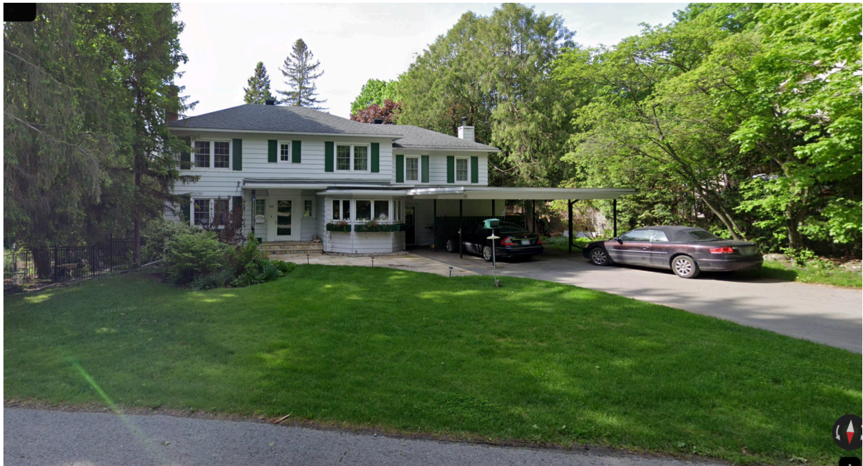
175 Juliana Road wide expansive front yard (13m) and wood siding. Google street view
