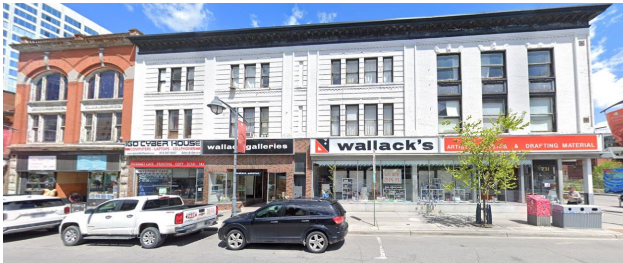
Figure 14: The painted brick commercial range 223-231 occupies the southern half of the block with the Wallacks Art Supply wrapping around the corner and extending along Lisgar Street.
