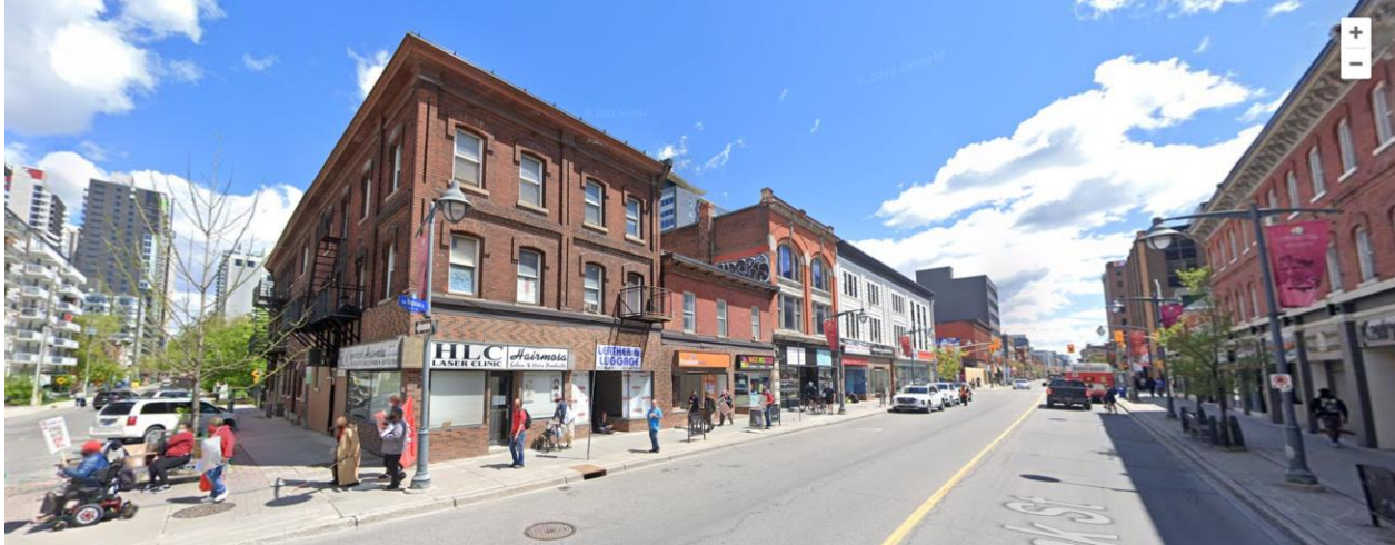
Figure 7: Street view of the properties looking south-east.
