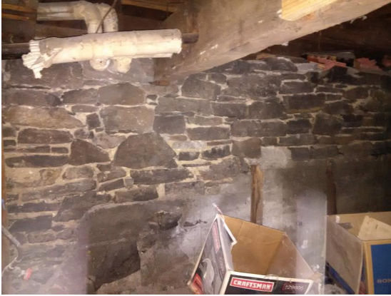
Photo Four – Rubble Stone Wall
