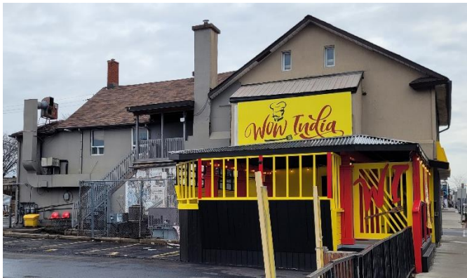
159 Montréal Road, west facade, mural visible, Source: City of Ottawa, 2024
