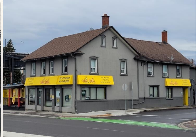
159 Montréal Road east façade, Source: City of Ottawa, 2024
