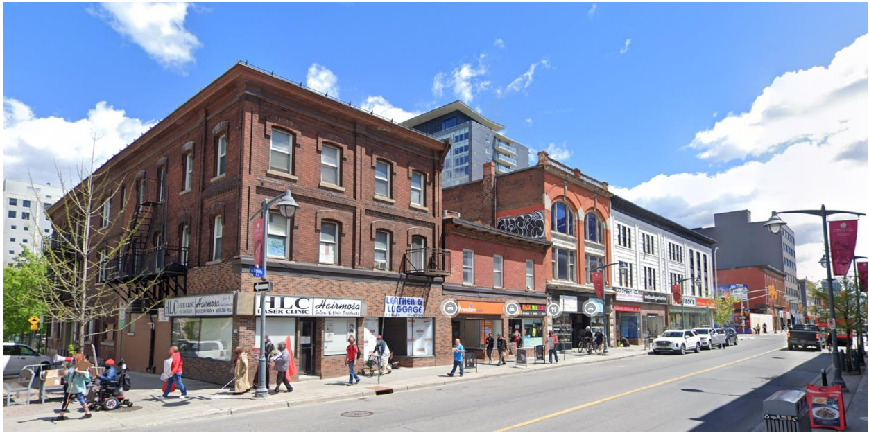
Bank Street looking south
