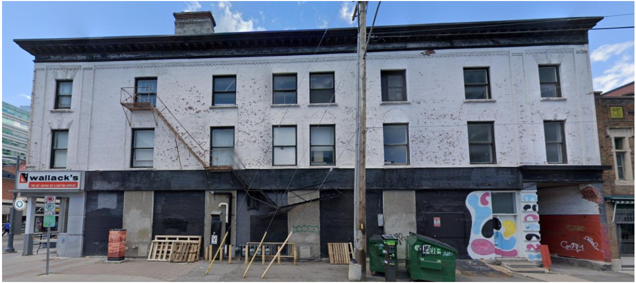
South façade of 223 Bank Street
