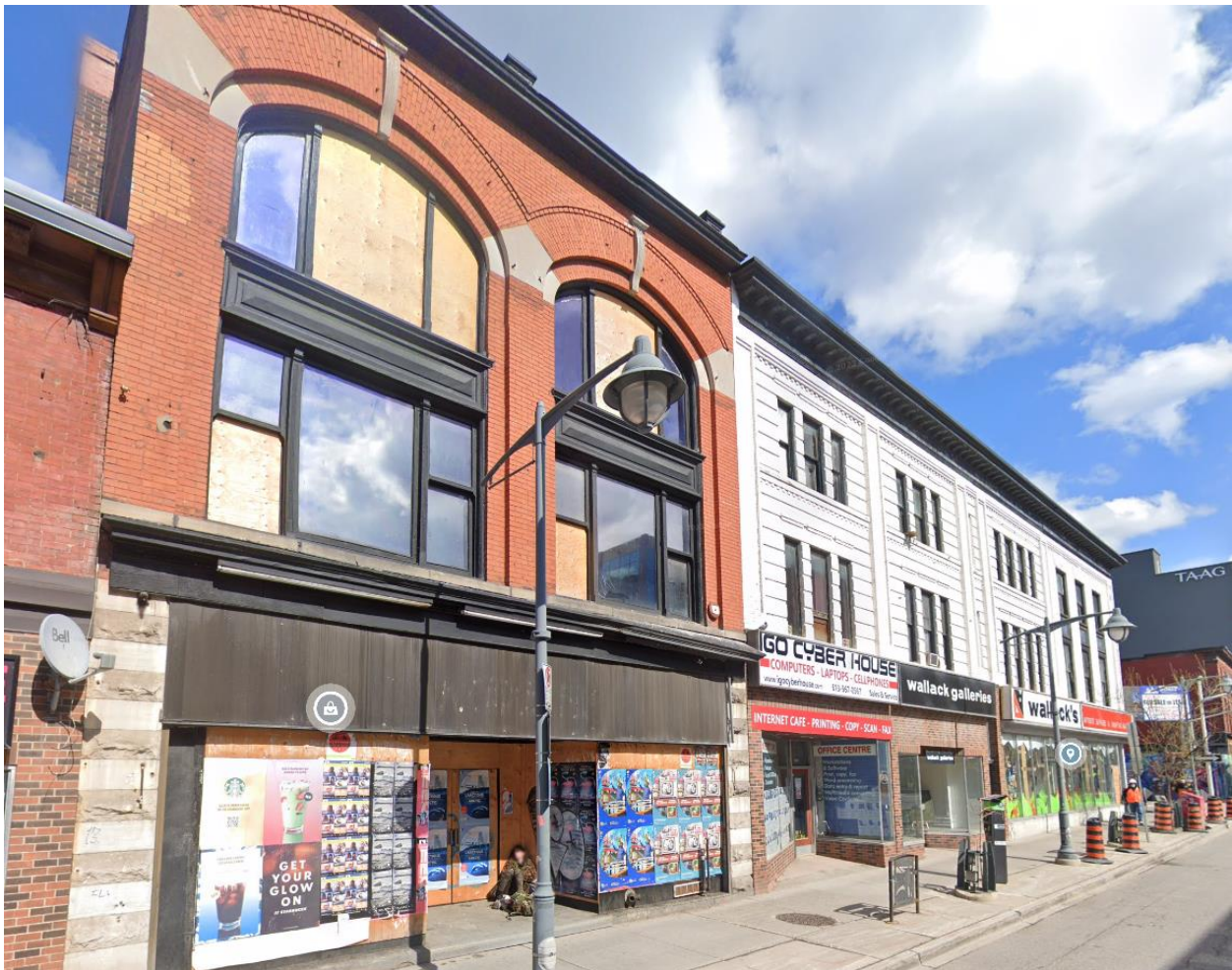
West façade (Bank Street) of 219-223 Bank Street
