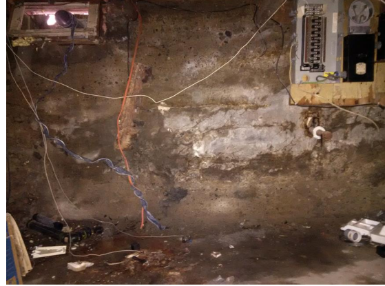
Photo Five – Underpinning/Remediation
