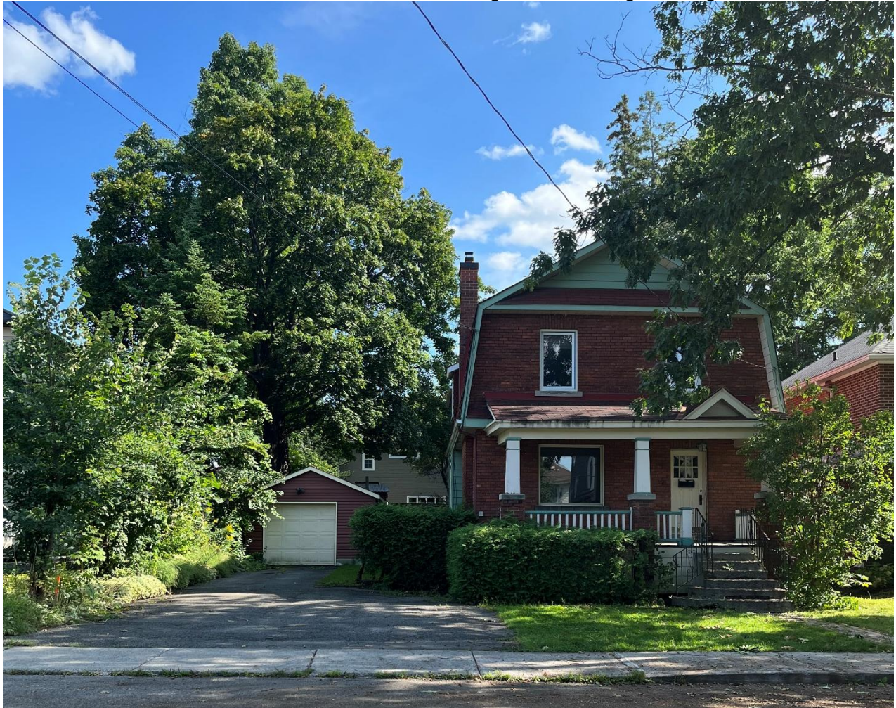
Figure 3: Existing Building on the Subject Site
