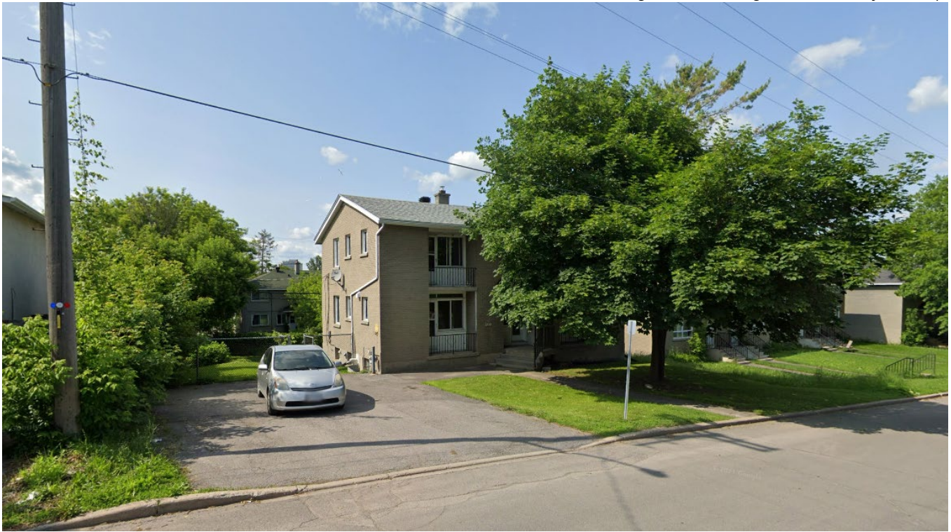
Figure 1: Existing home on Subject Property
