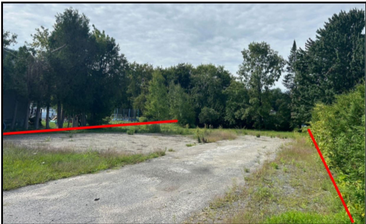
Image taken August 2024 showing the subject property after the 2023 fire.
