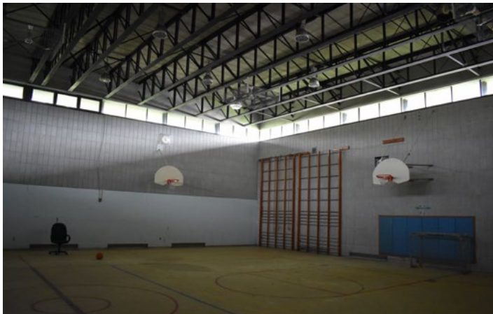
Figure 16. Building D, overall gymnasium view (ERA, 2021).
