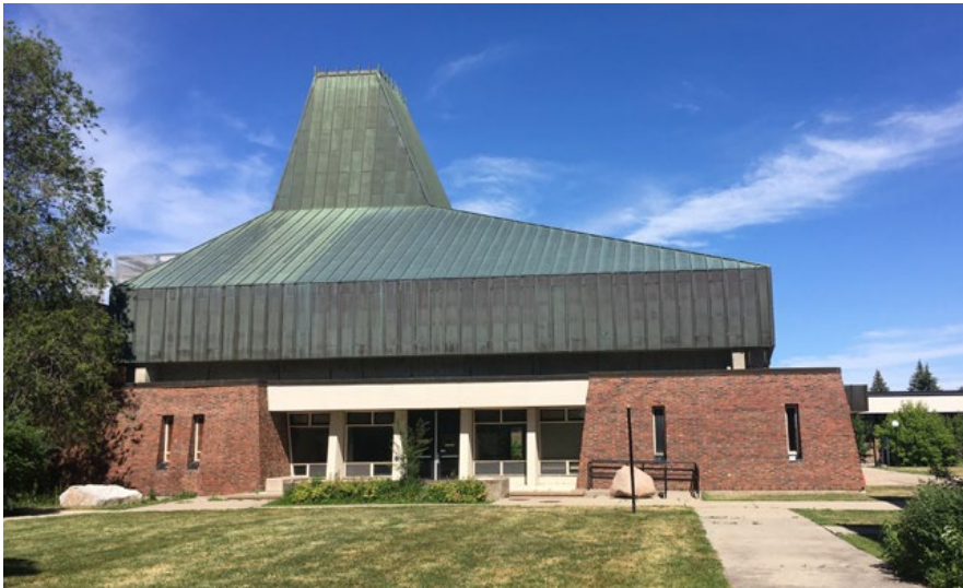
Figure 1. Building A, west elevation (ERA, 2021).
