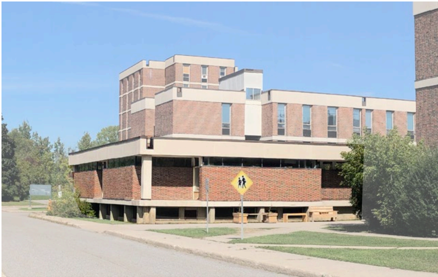
Figure 22. Building I viewed from southwest (ERA, 2021).
