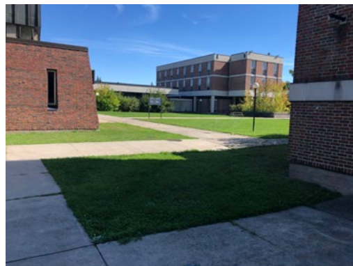
Exterior Circulation in Courtyards (ERA, 2021)
