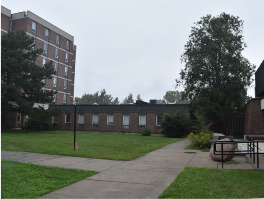
Figure 8. Building B, from Sisters' courtyard (ERA, 2021)
