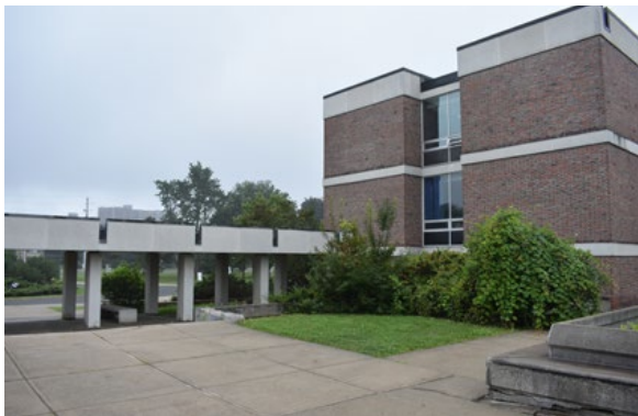
Figure 32. Existing conditions at main entrance (ERA, 2021).
