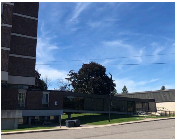
Figure 13. Connection to Building M (ERA, 2021).
