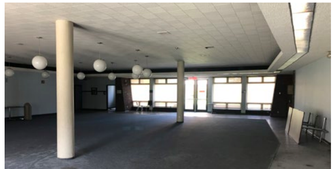
Figure 2. Building A, former cafeteria space at ground floor level (ERA, 2021).
