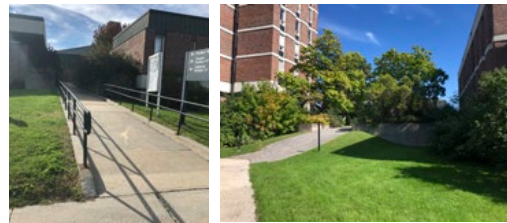
East Ramp and West Ramp (ERA, 2021)
