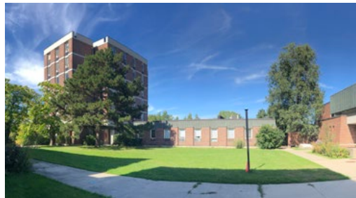
Secondary Courtyards (ERA, 2021)
