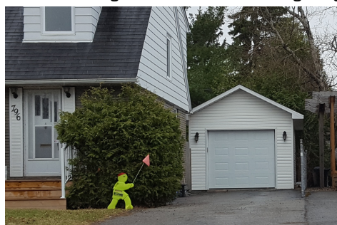
796 Wingate - rear detached garage
