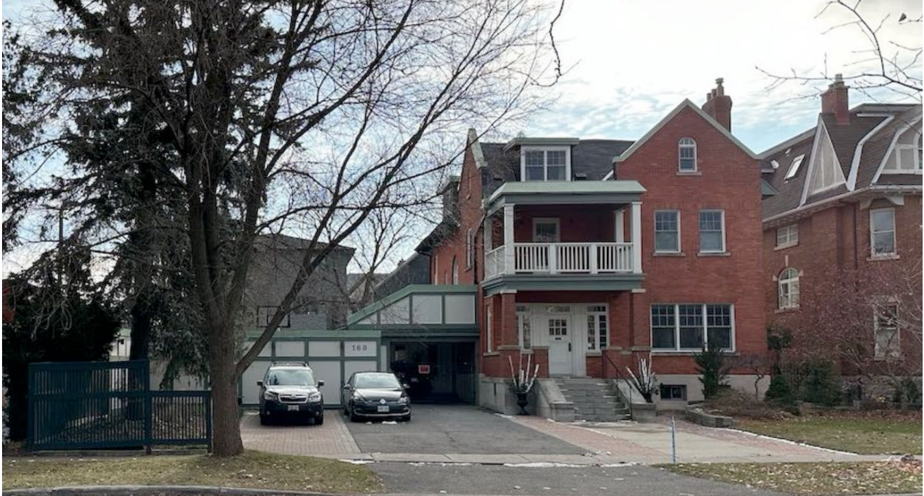
Figure 2: Street-view of the subject property.
