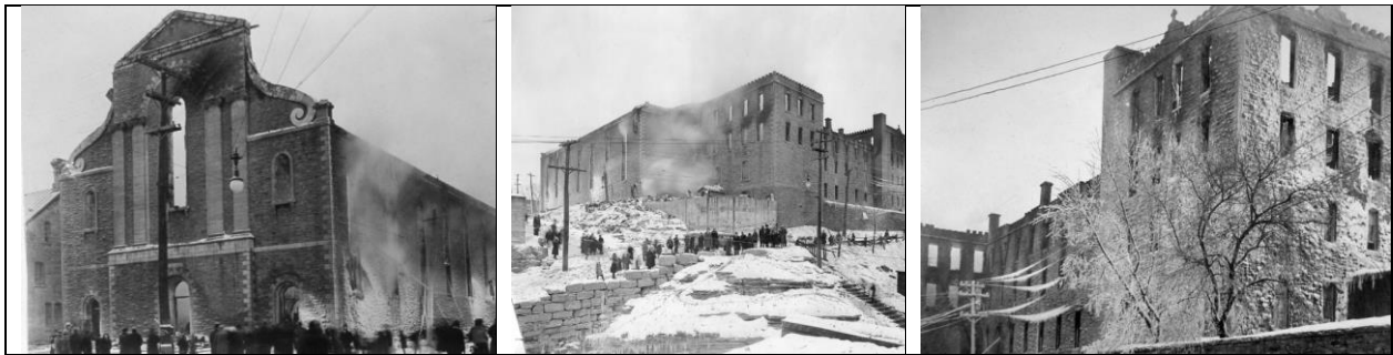
Figure 7: Views of the gutted church, 1899 wing, and the rectory following the 1931 fire. Source: Dominican Archives, Montreal.
