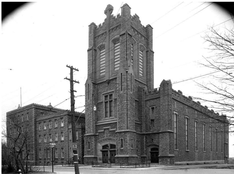
Figure 15: Post 1932 photo of the rebuilt church that was transformed with the introduction of a buttressed bell tower as part of the 1932 rebuild and a new rectory replacing the 1886 rectory after the February 1931 fire that gutted the church and portions of the monastic enclosure structures. Joseph Albert Larue the Dominican Architect was the architect for the 1932 rebuild. Alterations to the church included a new roof structure, new interior, bell tower, corner buttresses, window head alterations, and crenelated stone parapets. Source: Dominican Archives, Robert Smythe.
