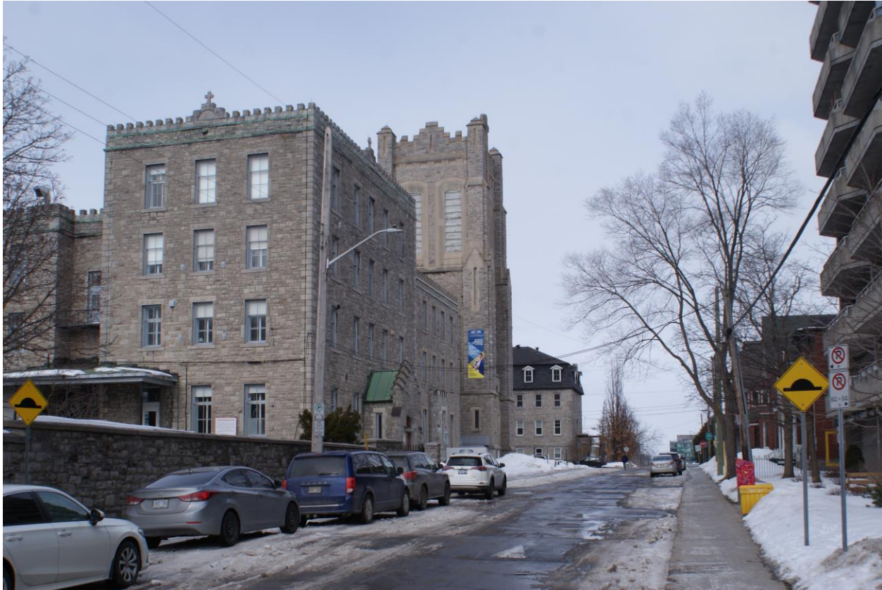
Figure 6: View north along Empress Avenue with the St. Jean Baptiste Convent and Church to the left with the Convent Notre Dame du Rosaire in the distance completed in 1890 to the design of Georges Bouillon, and the coop apartment residences (left) completed by the parish in 1975. Source: Commonwealth 2023
