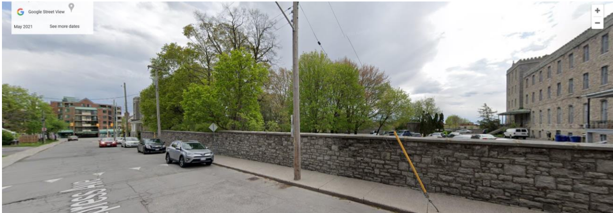
Figure 25 : A view along Empress with the stone wall and treed area associated with the seminary landscape. This bosch of trees is a remnant defining feature. Source Google Earth.
