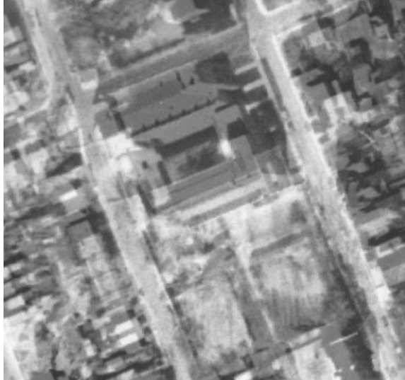
Figure 14: 1928 aerial view of the site at 90 Primrose and 96 Empress Avenue. Note the lack of a bell tower and the completed buildings that formed the monastic enclosure, although not extending to the south side of the church where the 1886 Rectory was located. A new rectory was completed as part of the 1932 rebuild designed by Joseph Albert Larue Architect for the Dominican Order. Note the landscape pattern to the south of the complex, with a cruciform path system illustrated in figure 12. The trees are limited to the edges of the property and what appears to be gardens, and a parking area. Source: Geotawa.
